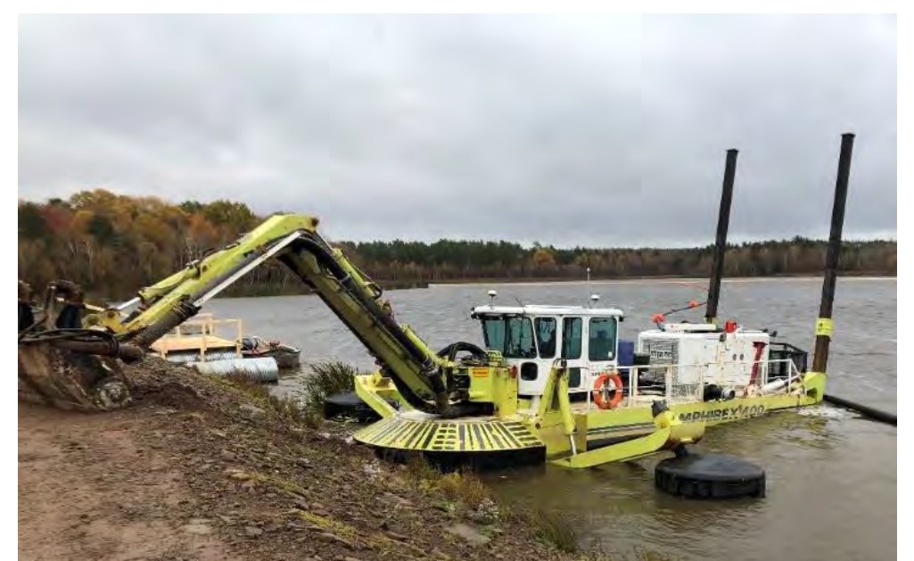
Removal in the Wet (Hydraulic Dredging)
