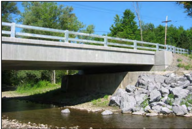
FC1 – Concrete Girder Bridge
