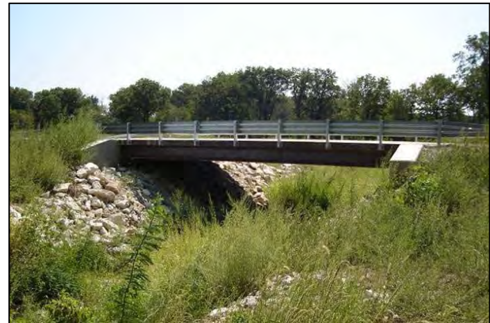
FC2 – Steel Girder Bridge
