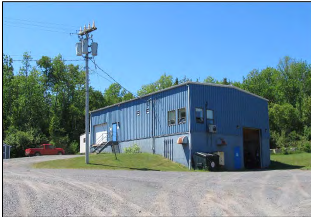
Permanent Buildings and Sheds
