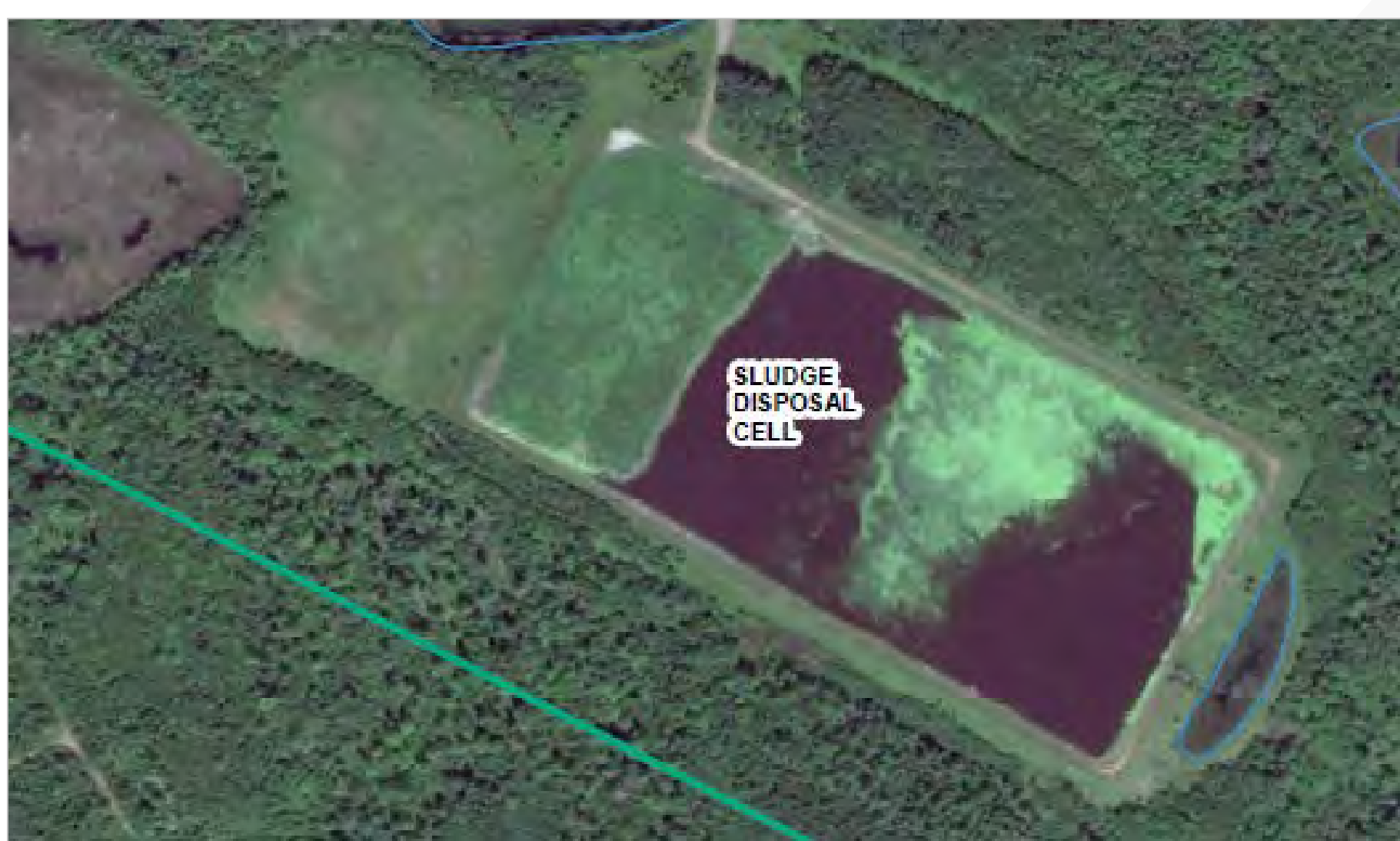
Existing Sludge Disposal Cell
