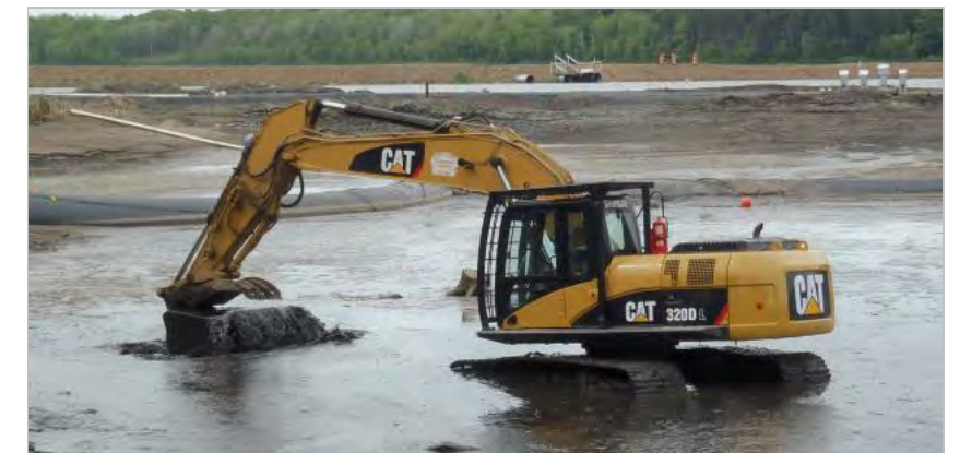
Dredging in the dry
