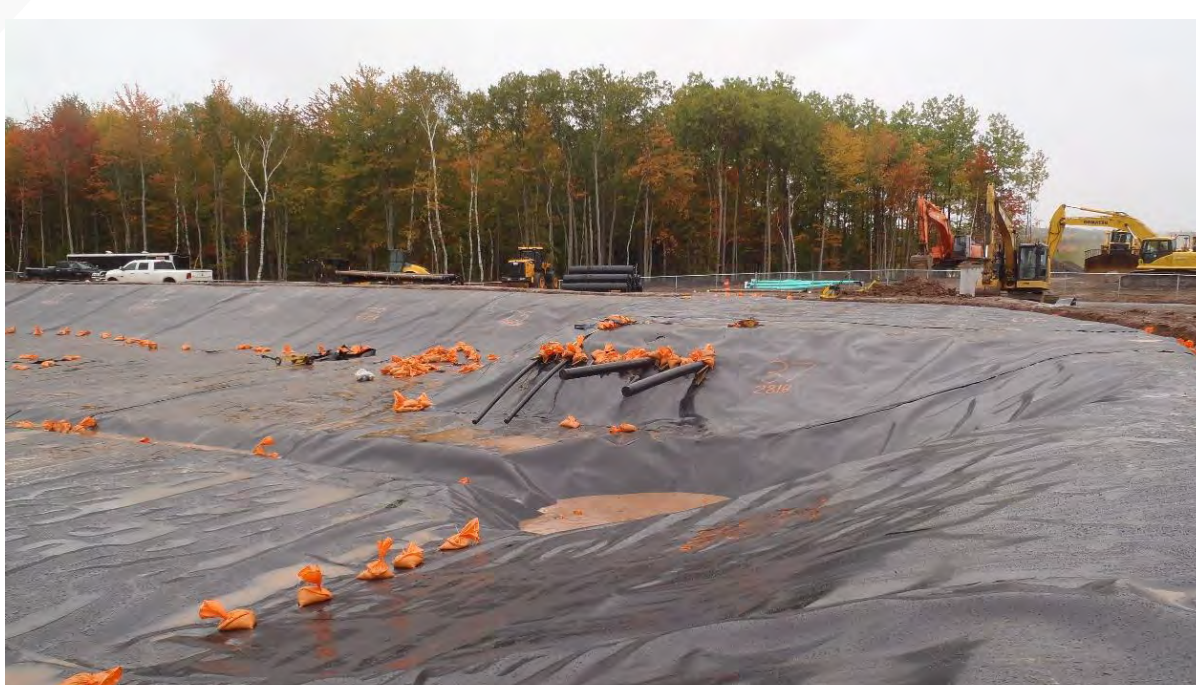
Treatment Pad Area
