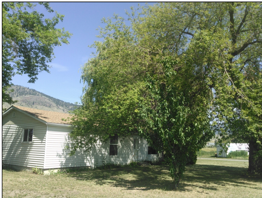
Photograph 2: Existing single-family home, located in the centre of the property. Photo taken facing North, July 17, 2018.
