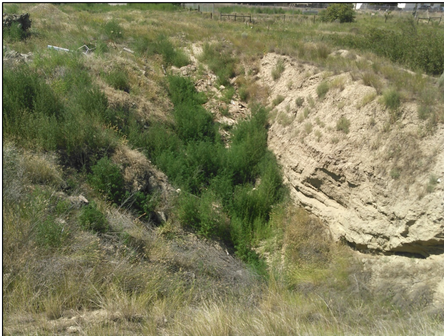
Photograph 4: Existing material debris pile, located along the northeastern Site perimeter. Photo taken facing northeast, July 17, 2018.
