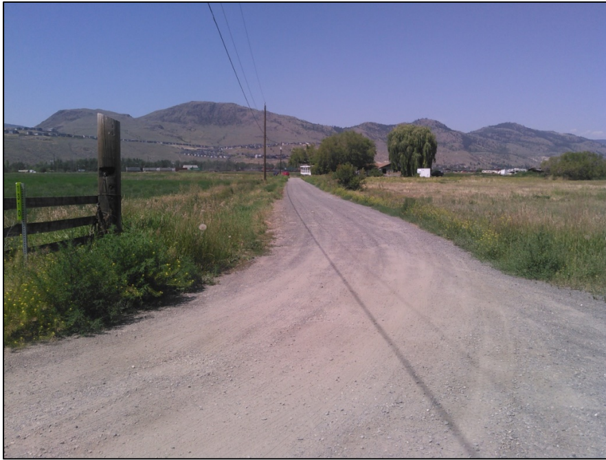
Photograph 7: Existing access road. Photo taken facing west, July 17, 2018.
