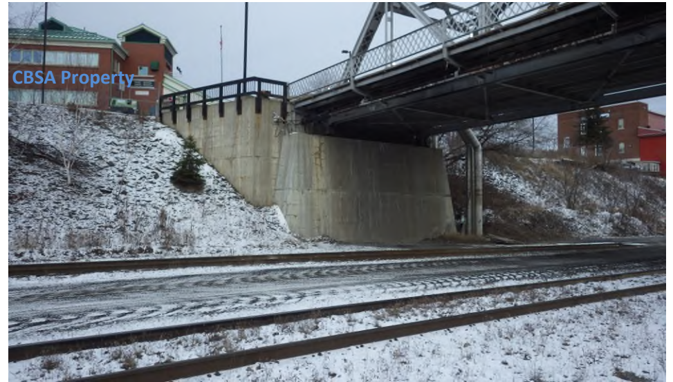
Northern river bank and abutment of existing bridge
