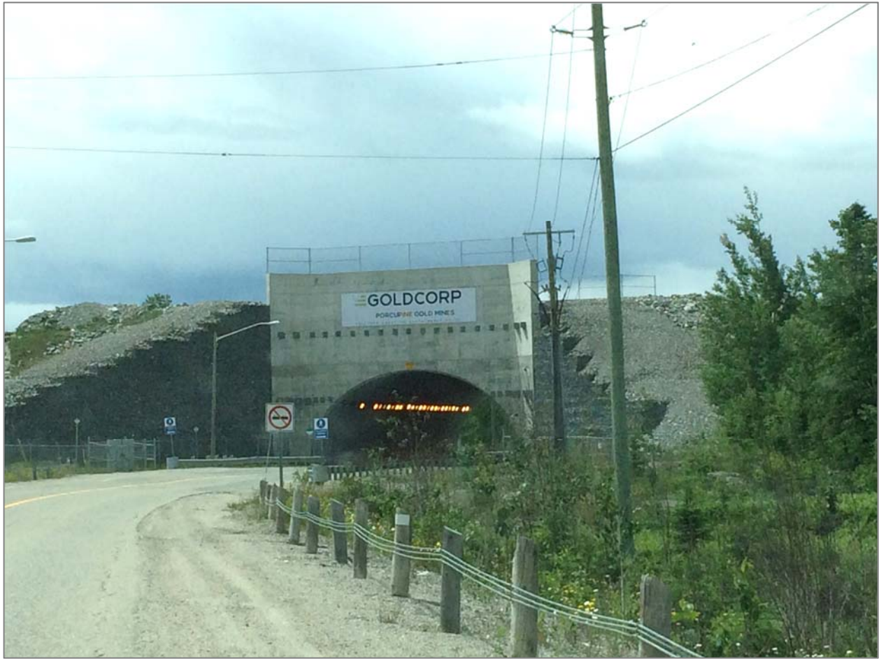
Plate 12: Gold Mine Road at Hollinger Haul Road Overpass looking northeast
