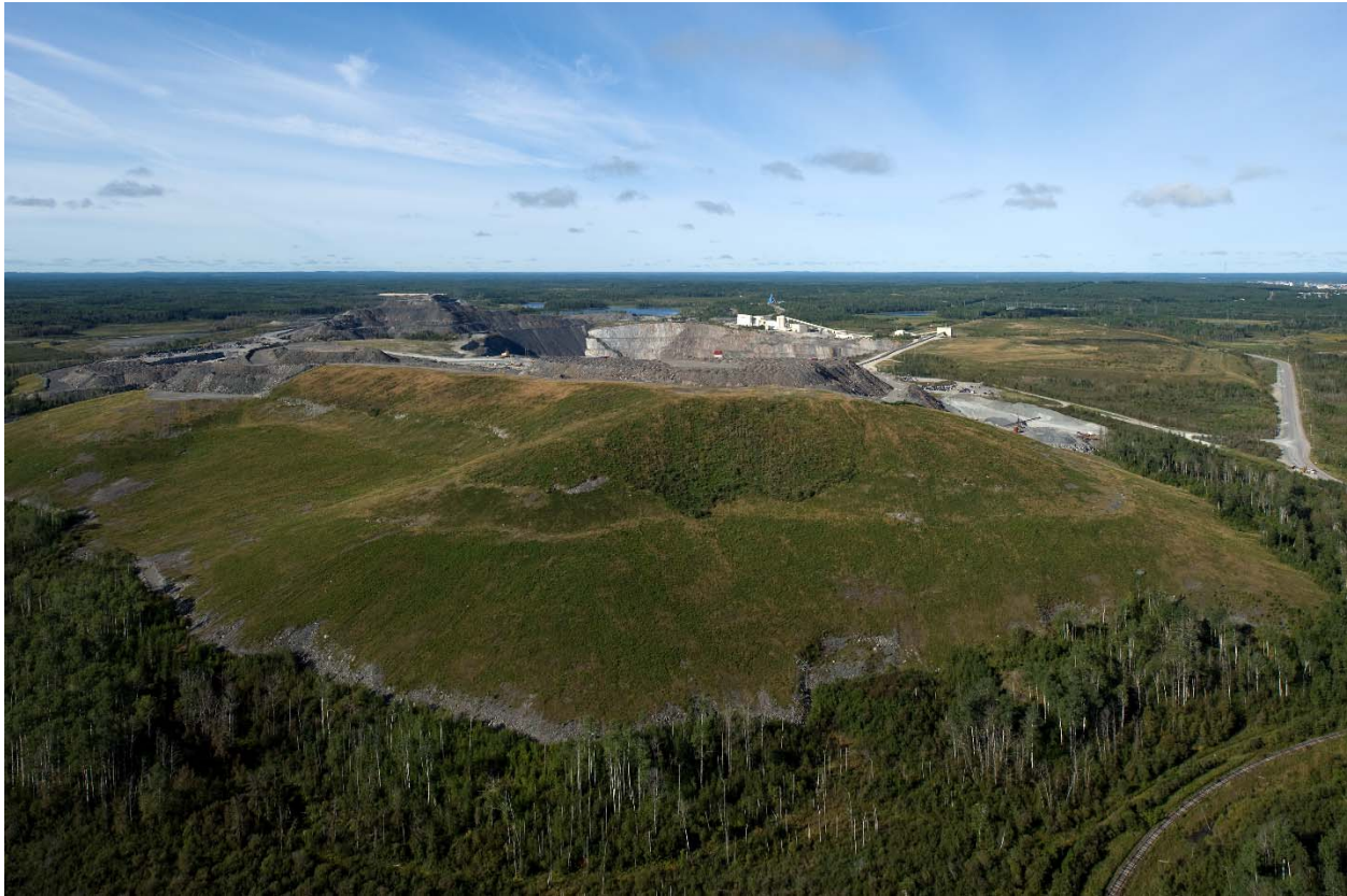
Plate 4: Reclaimed East Waste Rock Stockpile looking northwest (Dome Open Pit, Dome Processing Plant and Gold Mine Road in background)
