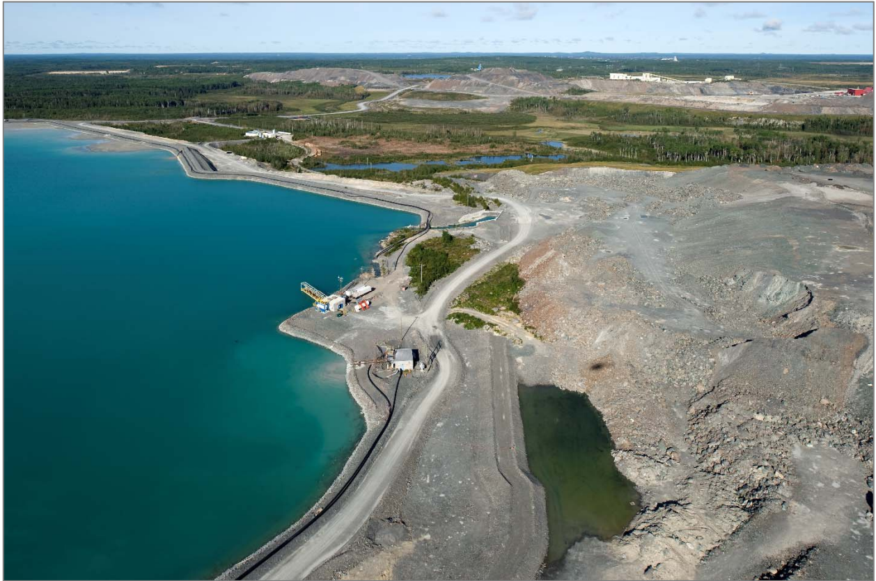
Plate 6: Dome TMA No. 6 (north dam), Effluent Treatment Plant and South Waste Rock Stockpile looking northwest (South Porcupine River and main Dome site in background)
