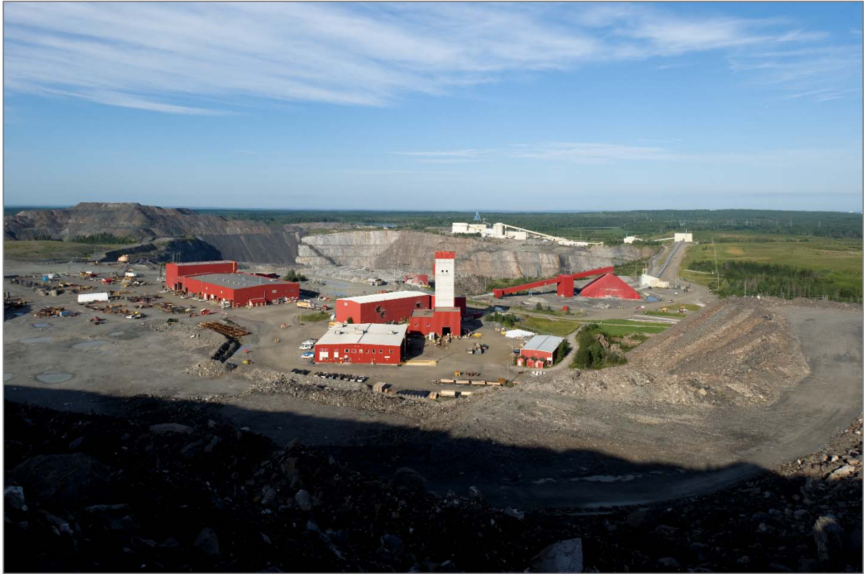
Plate 2: Dome Administrative / Crusher Complex looking southwest (Dome Open Pit and Dome Processing Plant in background)
