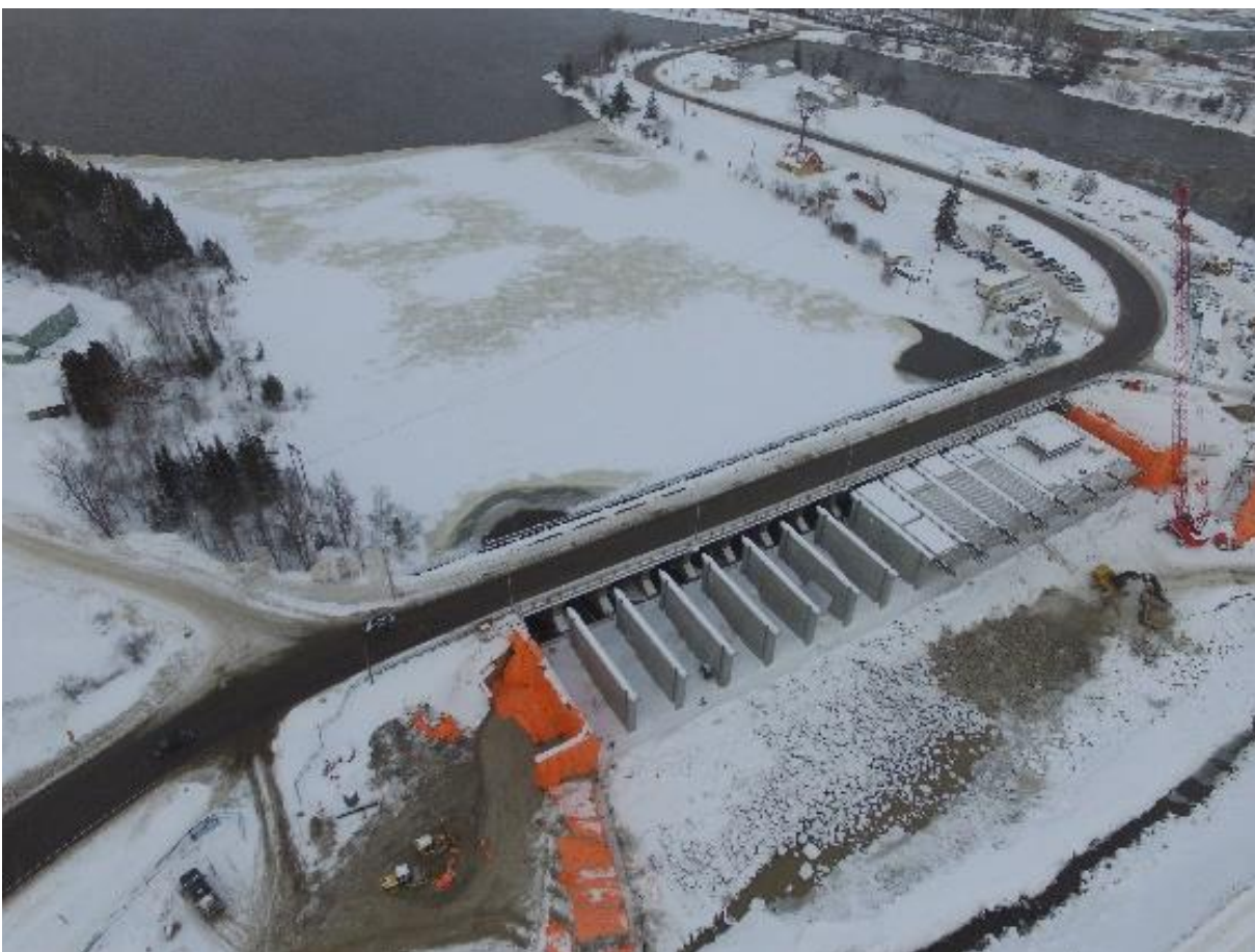
Photo 11.6 Example of the Formation of Ice Cover Upstream from the Dam on the Ontario Side During Reconstruction Work due to Reduced Current Velocities. On the Right, we see the Quebec Side Completely Ice-free.
