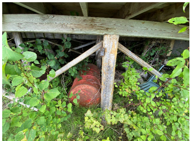
Plate 4-12: Dimensional Lumber and Wood Beam Cabin Supports
