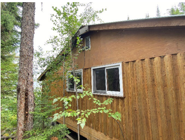
Plate 4-11: Side Fenestration and Wood Beam Wall Construction
