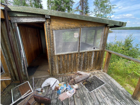
Plate 4-7: Cabin Porch and Entranceway
