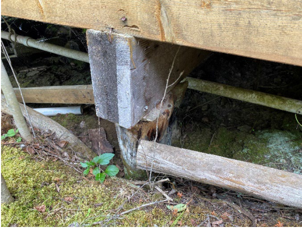
Plate 4-13: Cabin Floor Joists
