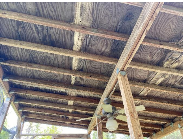
Plate 24: Roof Supports of Enclosed Front Porch
