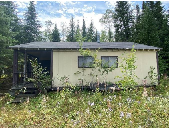
Plate 7: South (front) Elevation of the Cabin
