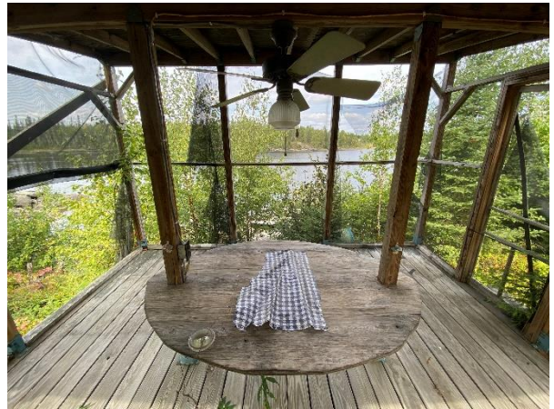
Plate 23: Interior of Enclosed Front Porch
