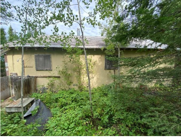
Plate 9: North Elevation of the Cabin
