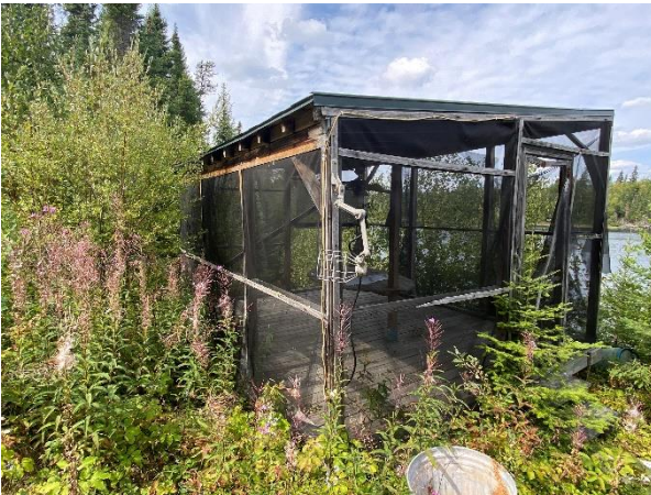
Plate 22: Enclosed Front Porch
