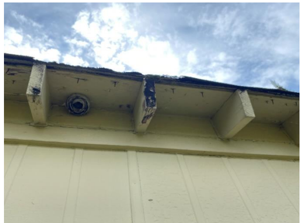
Plate 14: Protruding Rafters
