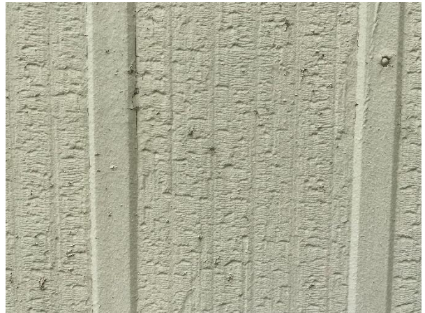
Plate 12: Board and Batten Exterior Cladding
