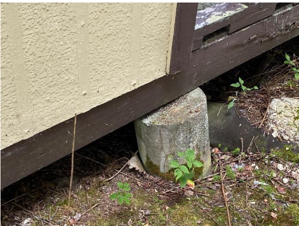
Plate 19: Concrete Foundational Supports
