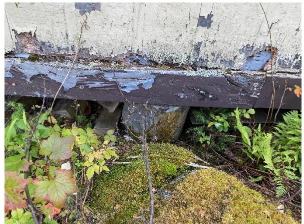
Plate 20: Concrete Foundational Supports
