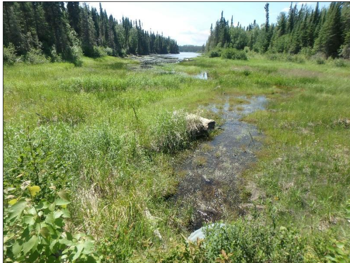
Facing downstream at culvert (Jul. 16, 2019)
