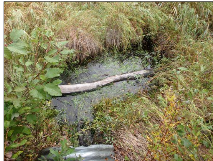
Culvert inflow (Sep. 17, 2019)
