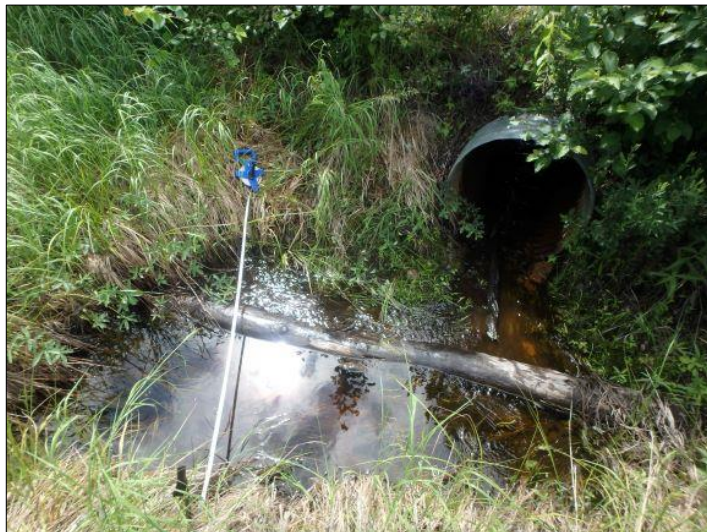
Culvert inflow (Jul. 20, 2019)
