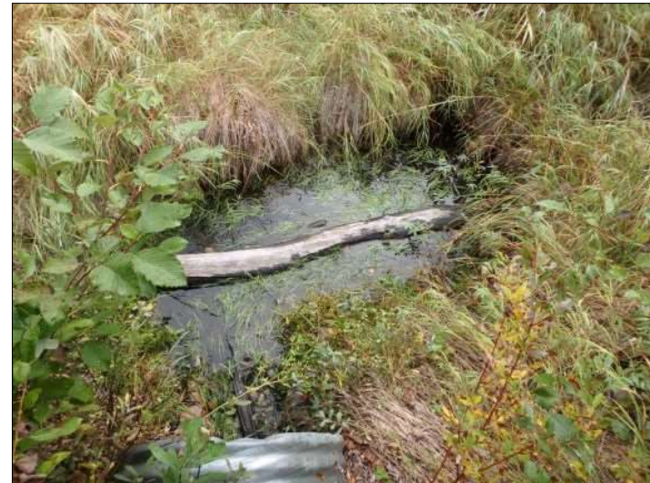
Culvert inflow (Sep. 17, 2019)
