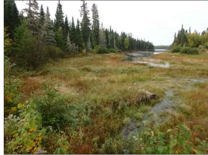
Facing downstream at culvert (Sep. 17, 2019)
