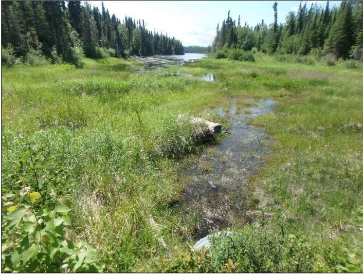
Facing downstream at culvert (Jul. 16, 2019)
