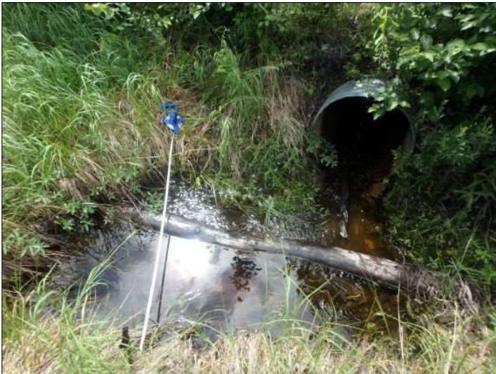
Culvert inflow (Jul. 20, 2019)
