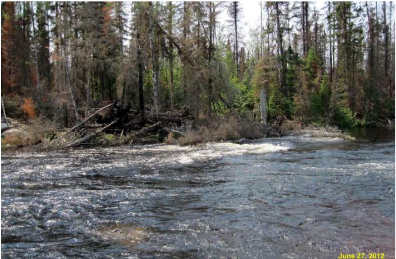
Figure E: View of Birch River Crossing – South Abutment
