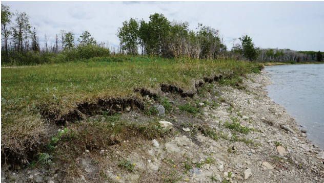
Photo Location DR12: looking downstream
