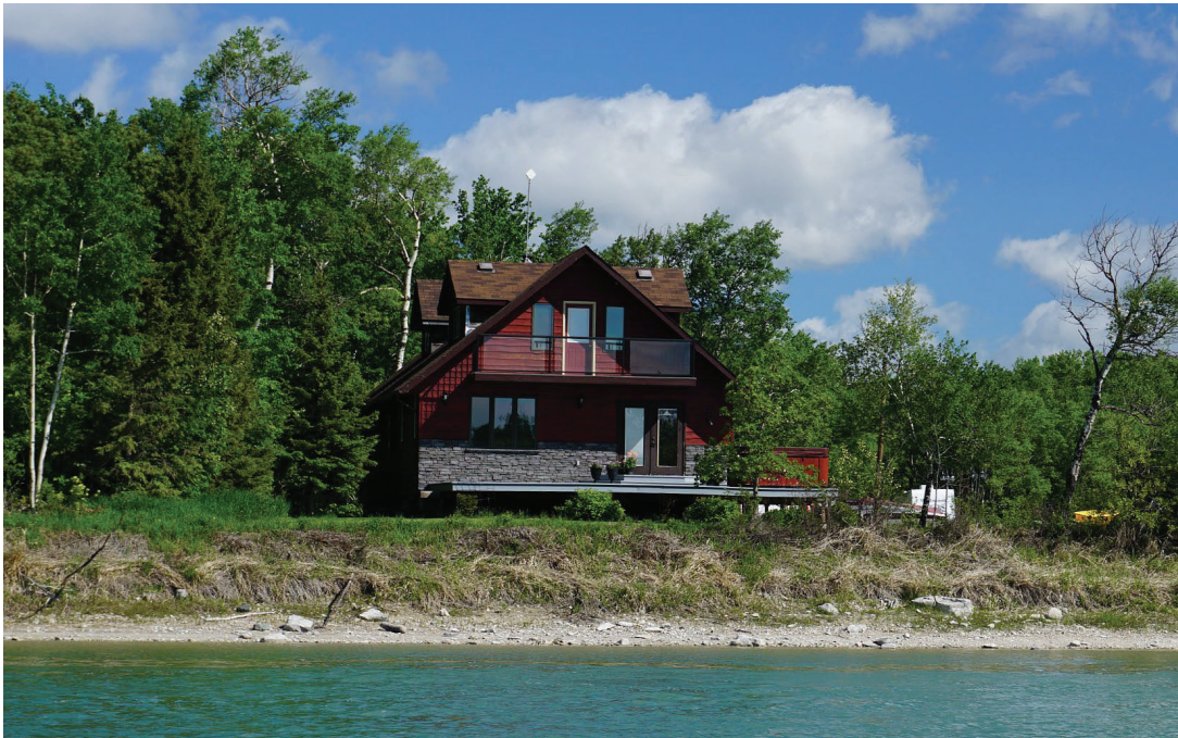
FIGURE 56: ERODING RIVERBANK IN FRONT OF HOME (DOWNSTREAM OF SITE J), JUNE 11, 2019
