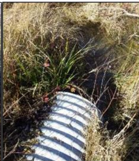
Figure B-5. Upstream (left) and downstream (right) views of Culvert 3C. The upstream side was blocked by debris and vegetation; blockage resulted in water flowing across the road.
