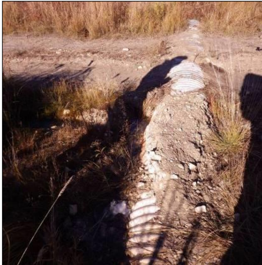
Figure 6. One of three culverts at Crossing 3, exposed across road and completely blocked at upstream end.
