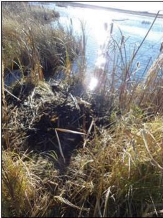
Figure C-16. Plugged culvert at Crossing 3.
