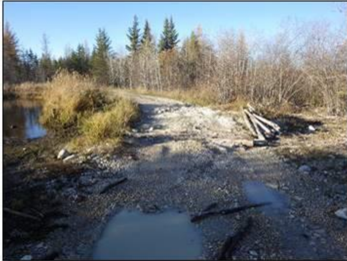
Figure C-7. Access road at Crossing 2. Road was washed out prior to clearing and grubbing of culvert.
