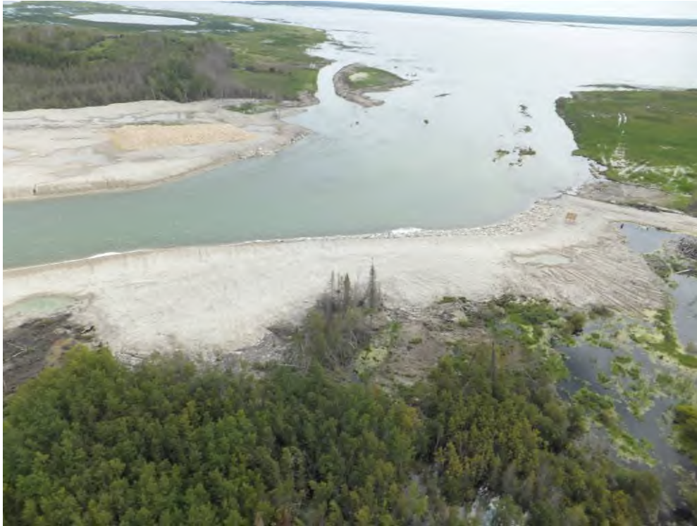
Photo 3 Reach 1 Emergency Channel Inlet
