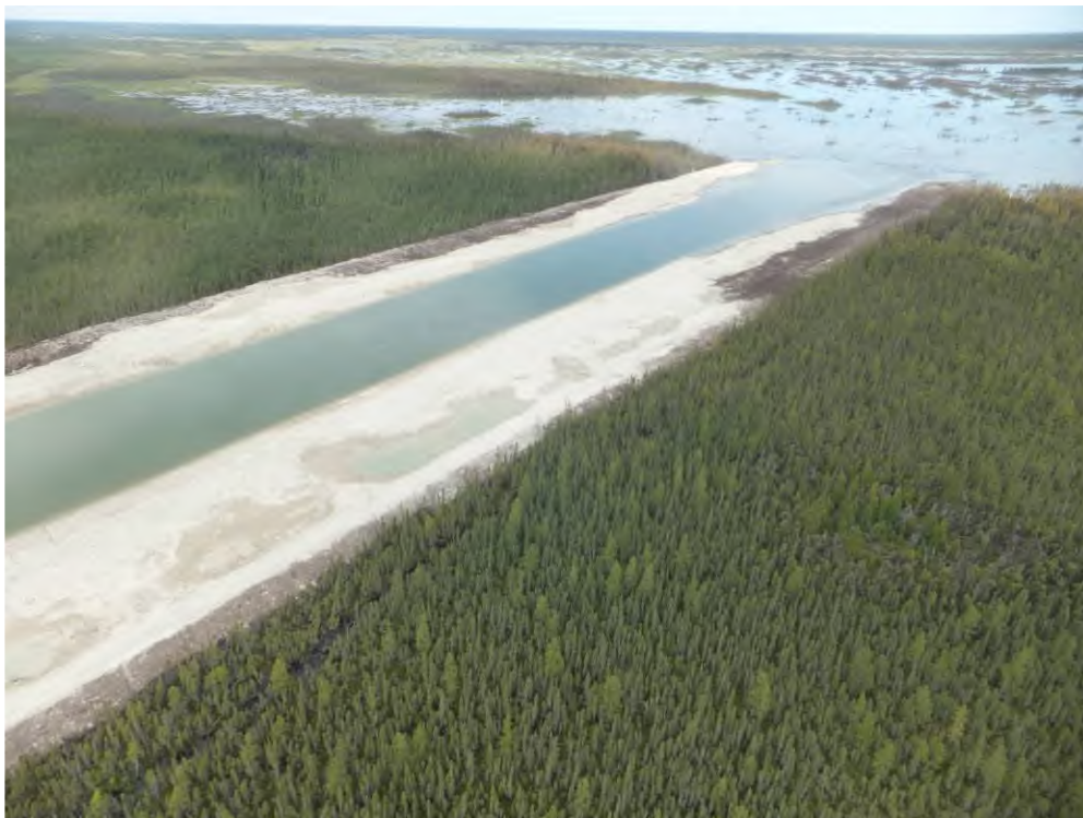
Photo 4 Reach 1 Emergency Channel Outlet
