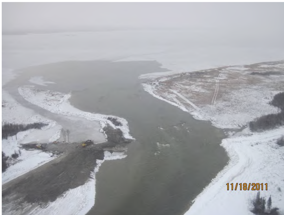
Photo 3 Reach 1 Emergency Channel Inlet
