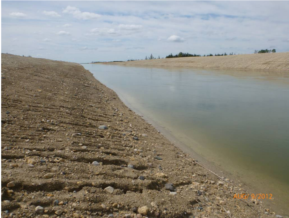
Photo 1 Reach 1 Emergency Channel Looking Upstream of Metering Location
