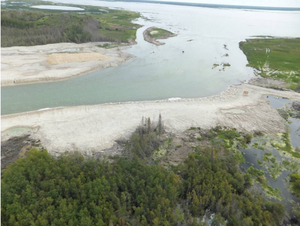
Photo 3 Reach 1 Emergency Channel Inlet
