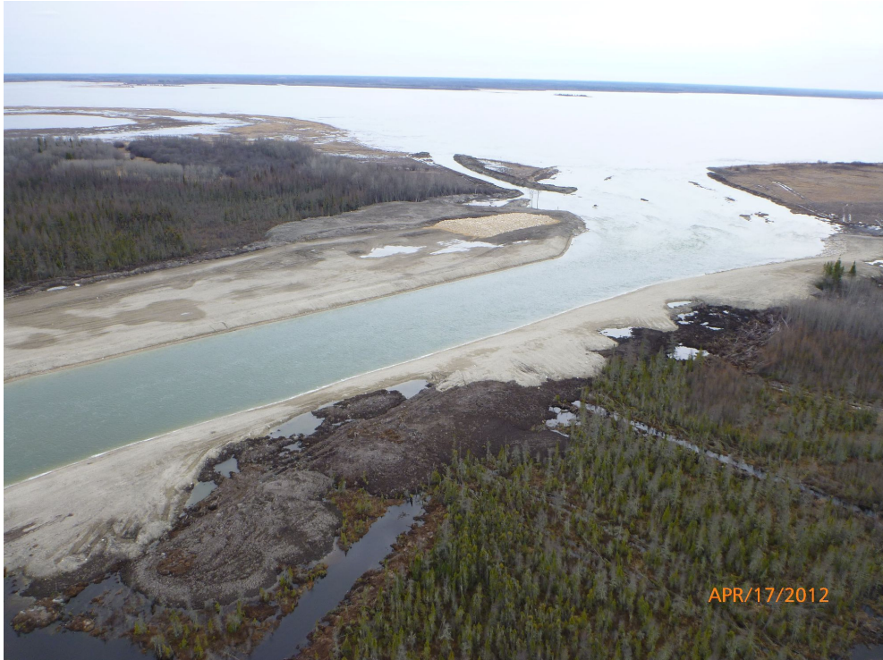
Photo 3 Reach 1 Emergency Channel Inlet
