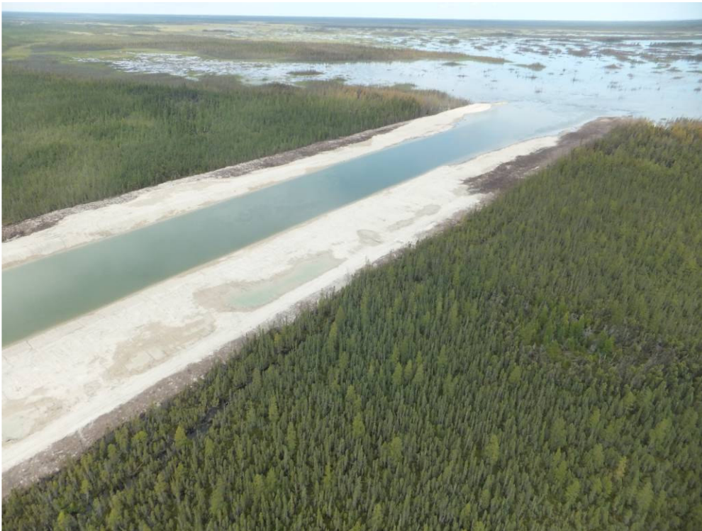
Photo 4 Reach 1 Emergency Channel Outlet
