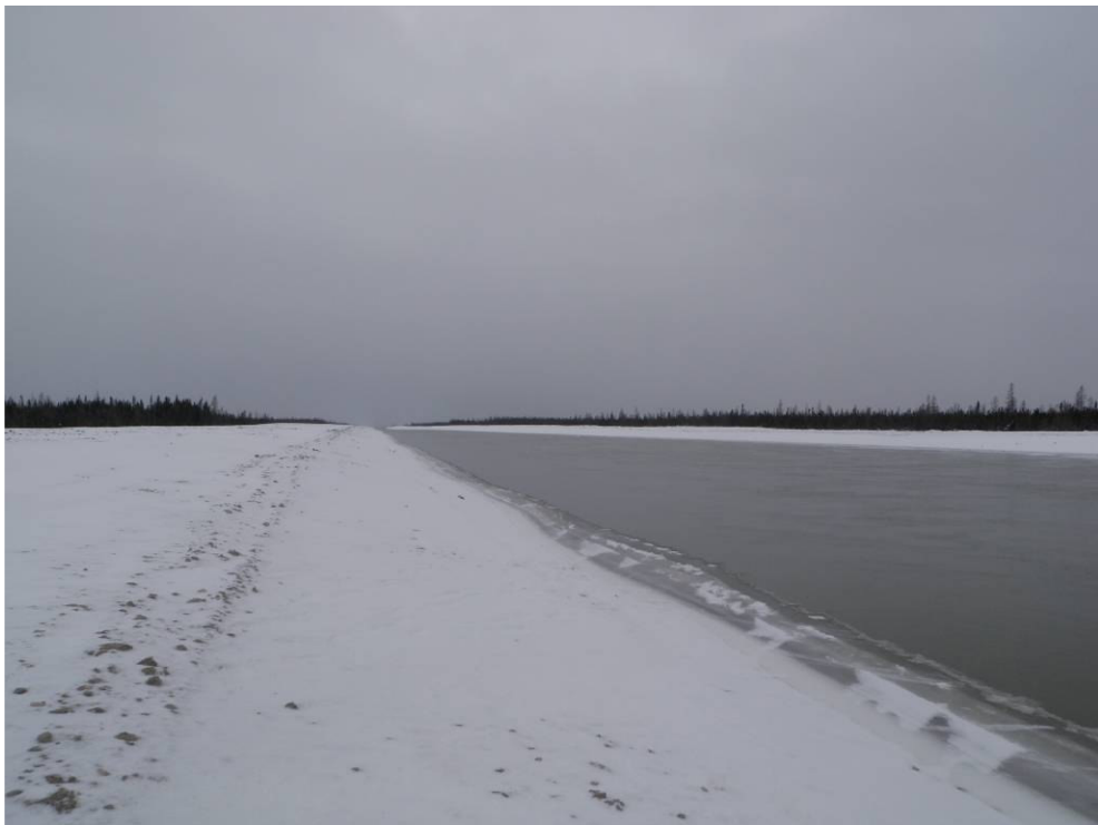
Photo 2 Reach 1 Emergency Channel Looking Upstream of Metering Location
