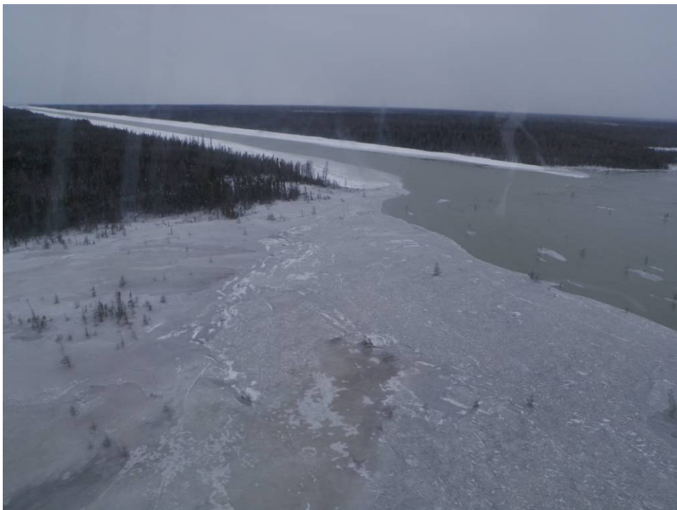
Photo 4 Reach 1 Emergency Channel Outlet
