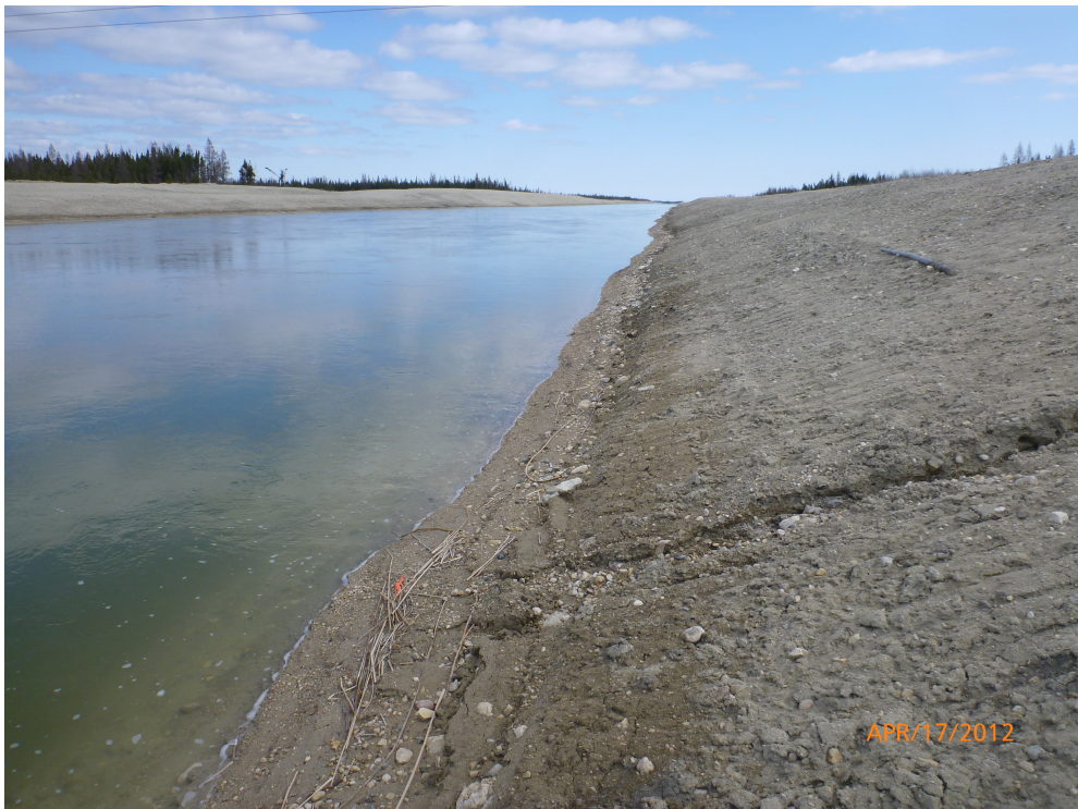
Photo 2 Reach 1 Emergency Channel Looking Downstream of Metering Location
