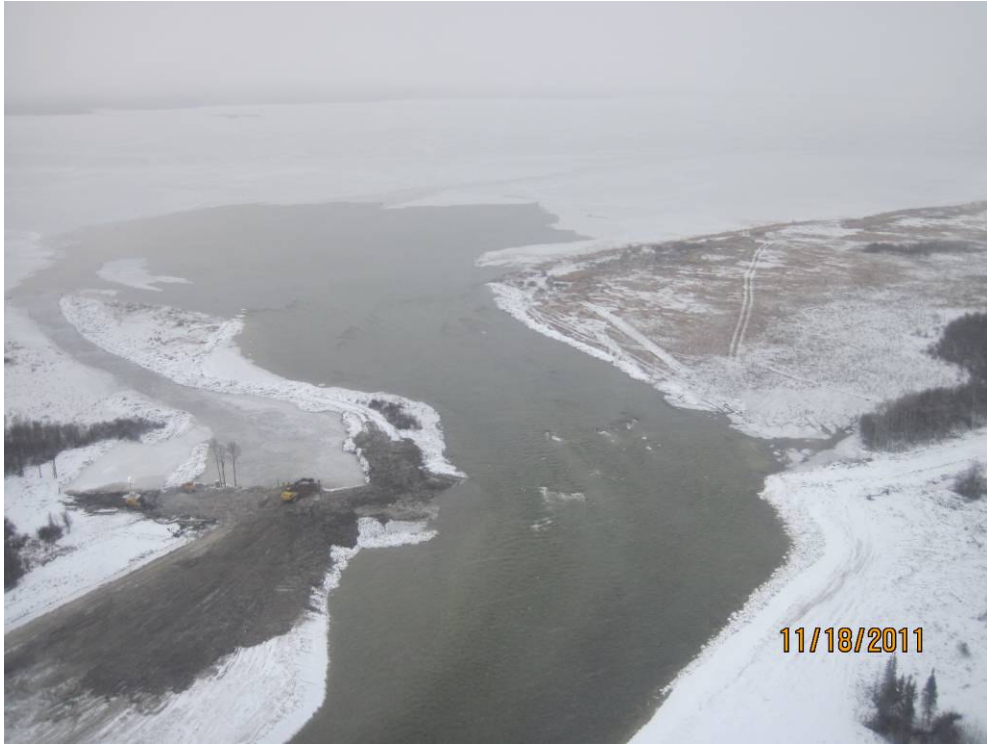
Photo 3 Reach 1 Emergency Channel Inlet
