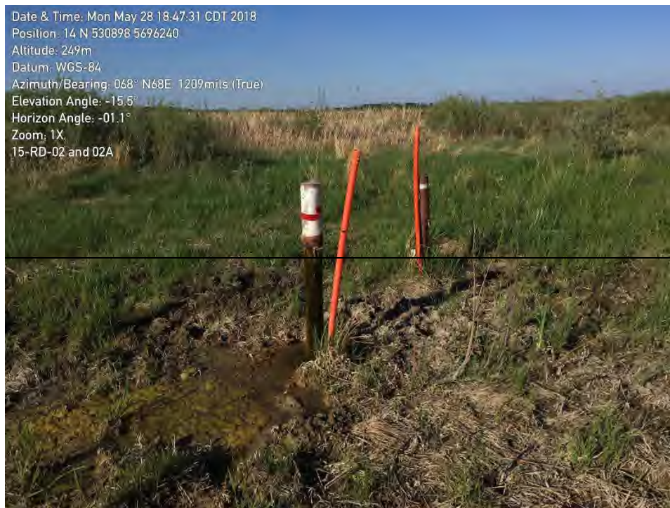
Figure 4: 15-RD-02, showing leaking casing and wet ground around well.
