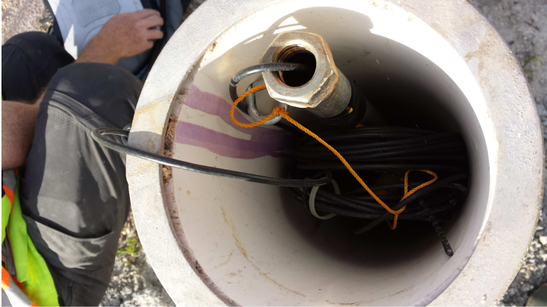
Photo 1. TH-EC-01WW2 – Showing packer, tubing and transducer installation.
