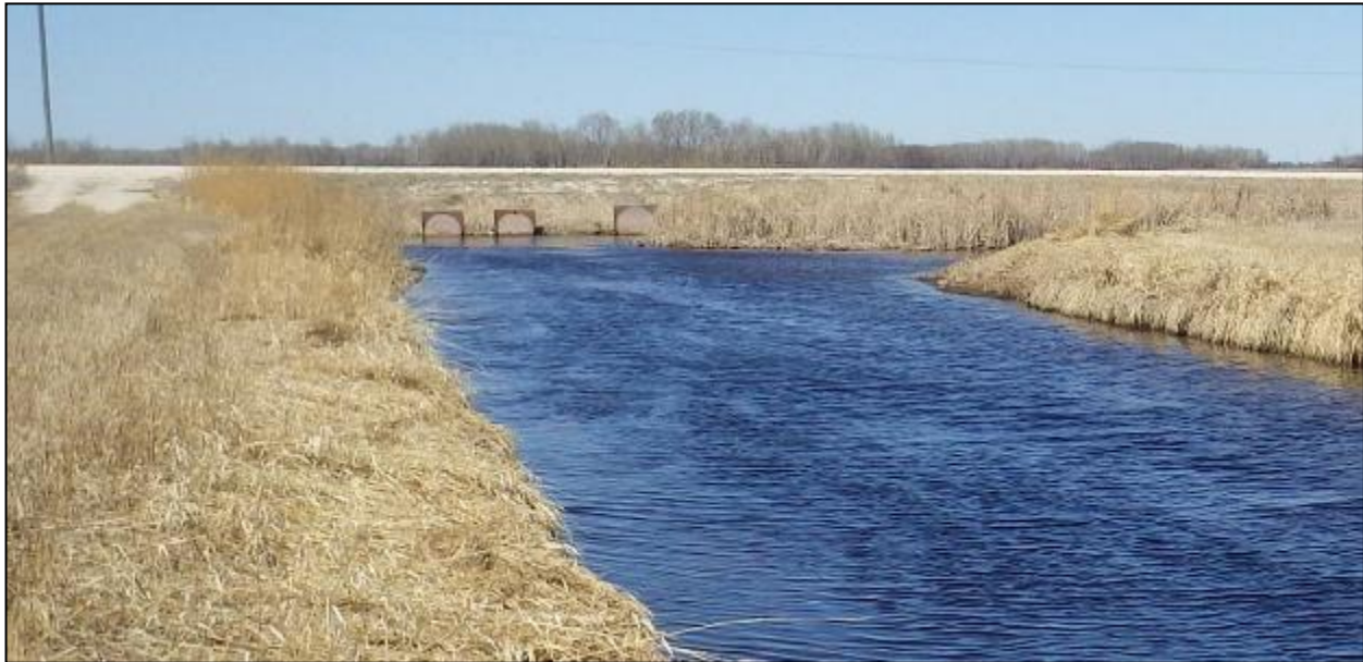
Figure 45. Facing upstream; Closed culverts at the downstream road crossing. The bypass drain enters from the right (east).
