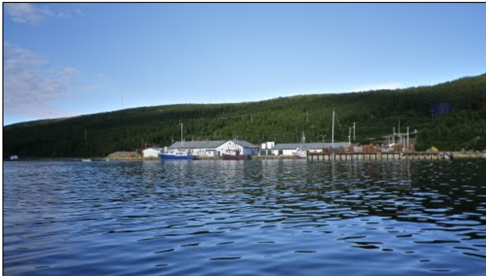
Photo 1 The port facilities in St. Lewis, NL.
