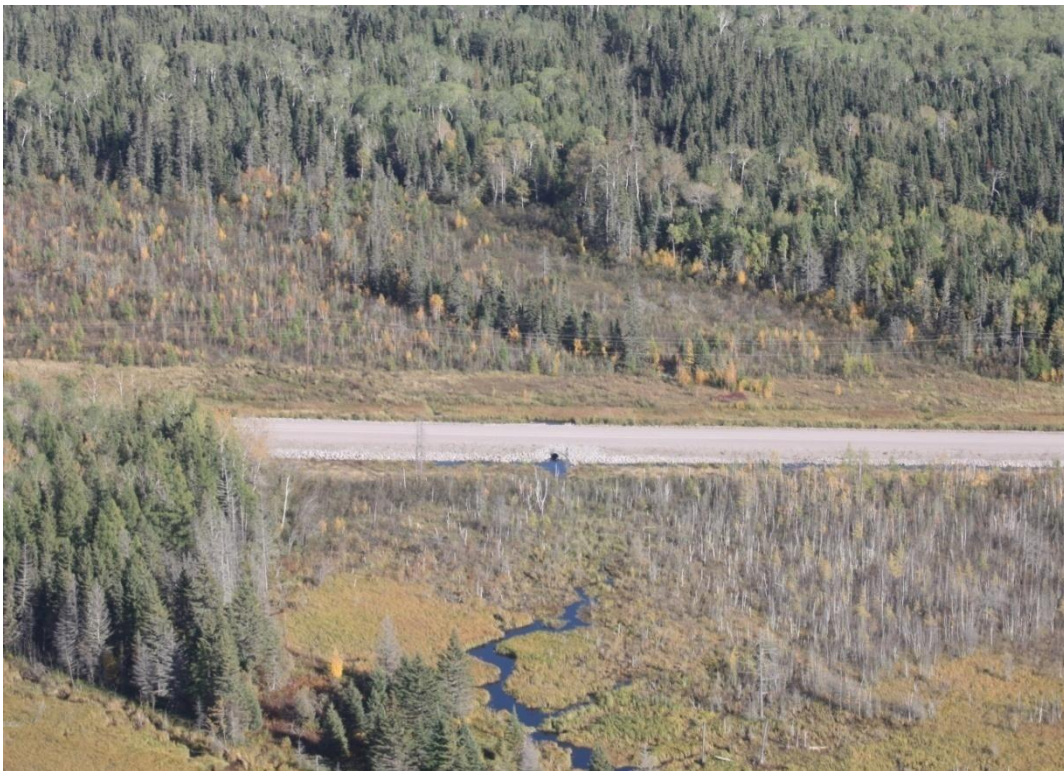
Photo 7: Small drainage/stream crossing – single culvert ( representative from P1 )
