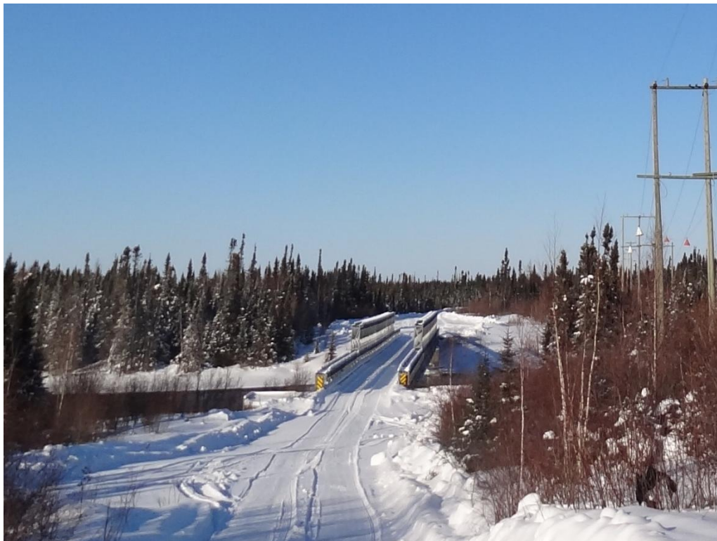
Photo 1: Existing single lane bridge crossing God's River to be replaced
