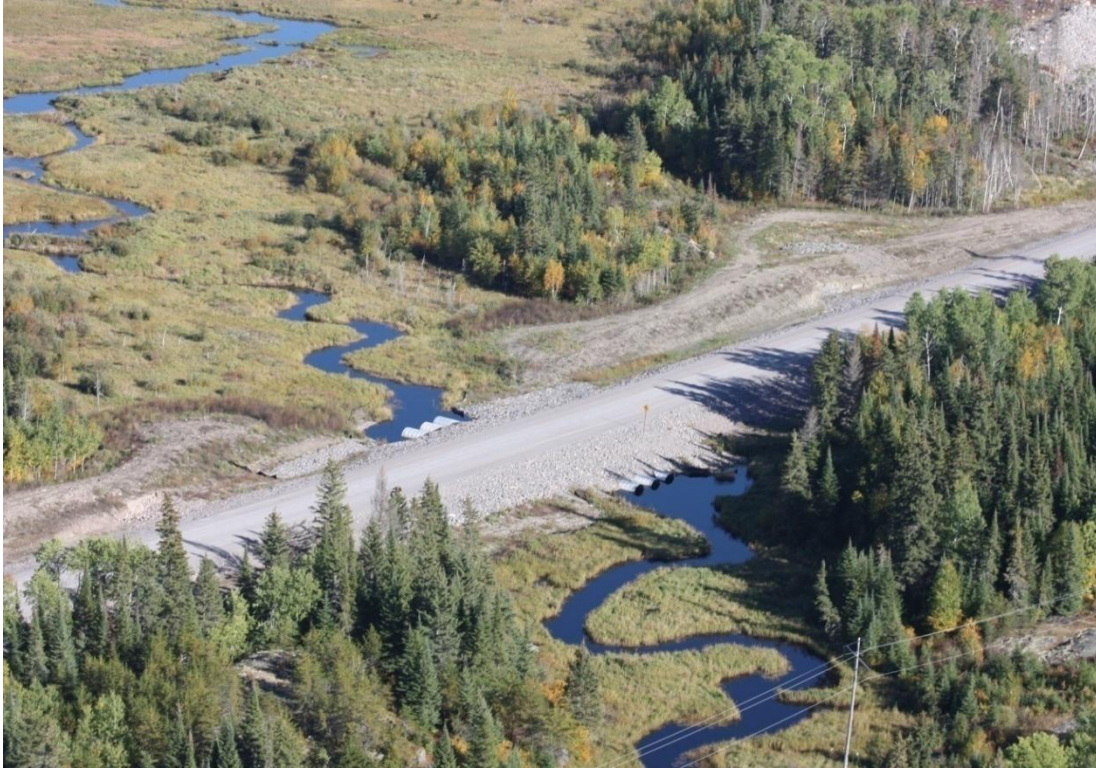
Photo 6: Stream crossing – three culverts ( representative from P1 )
