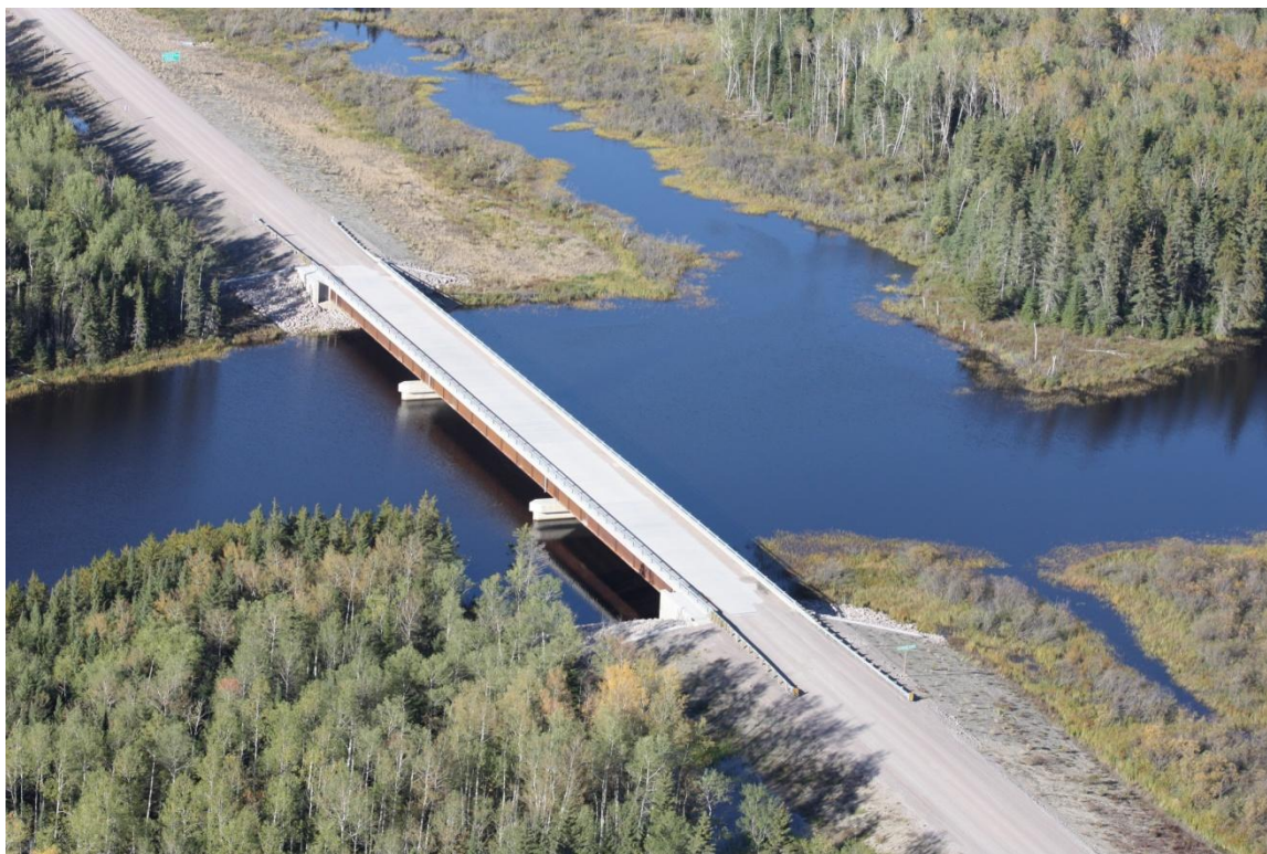
Photo 5: Stream crossing – bridge with piers over Longbody Creek ( representative from P1 )
