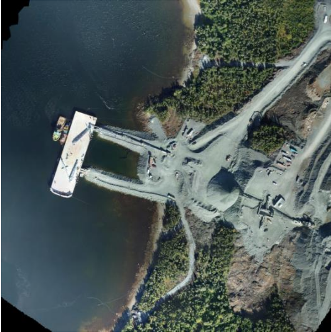
Photo 2: Dock configuration as constructed
