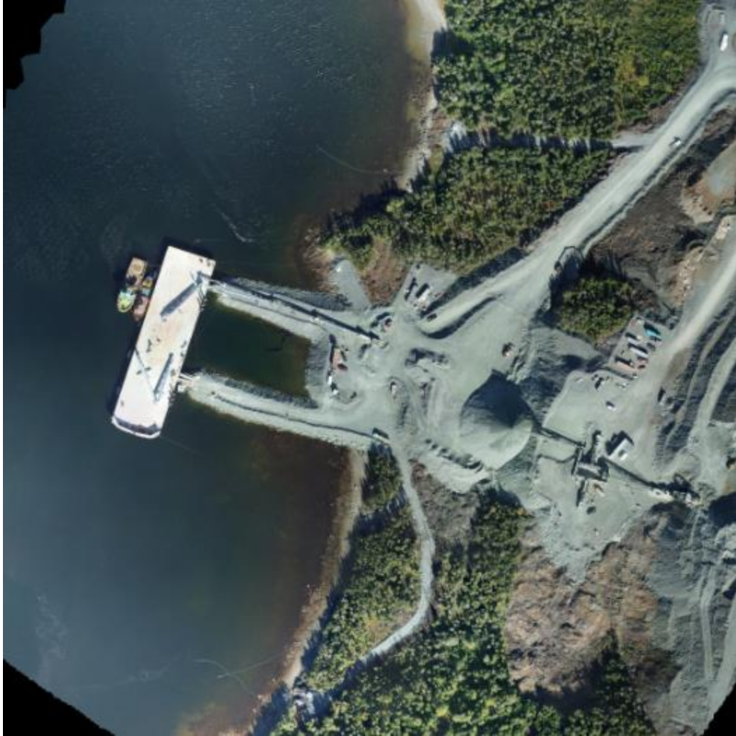
Photo 2: Dock configuration as constructed
