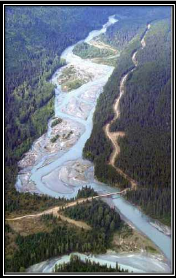
The Iskit River Bridge at the confluence of More Creek and the Iskit River
