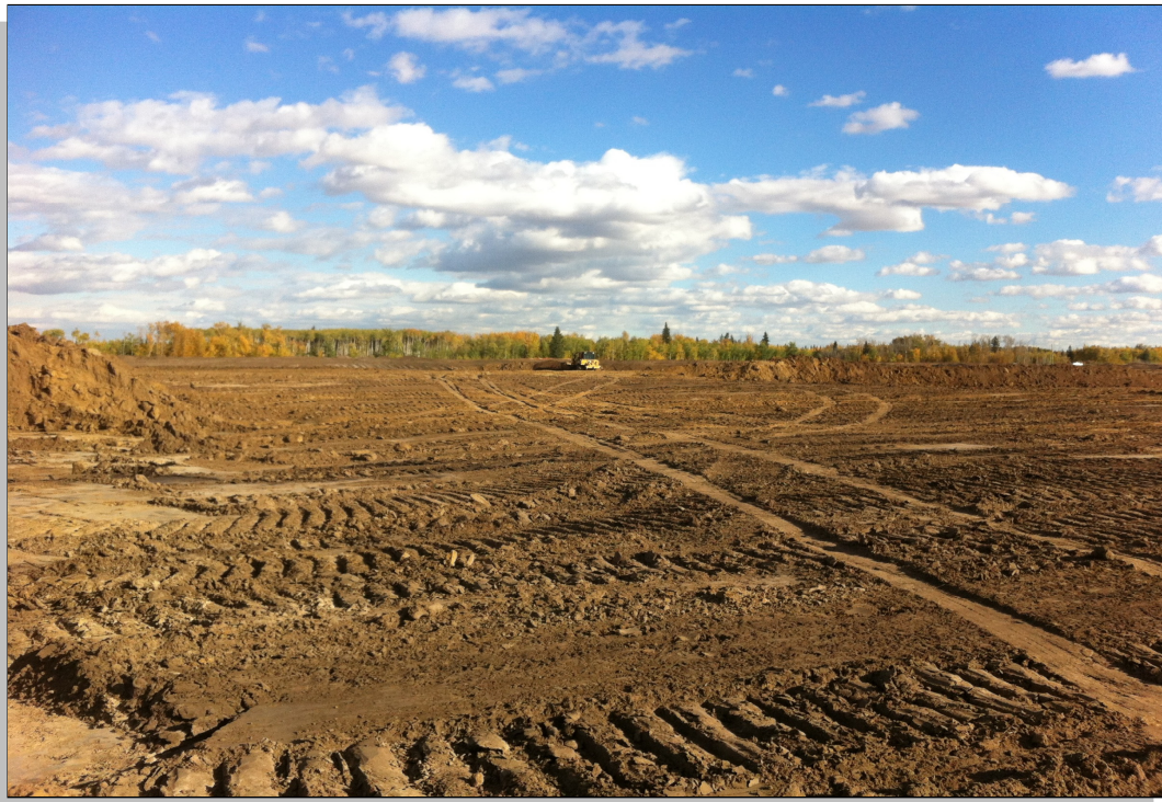
PHOTO 8: Alberta PDH Facility footprint during soil salvage.
