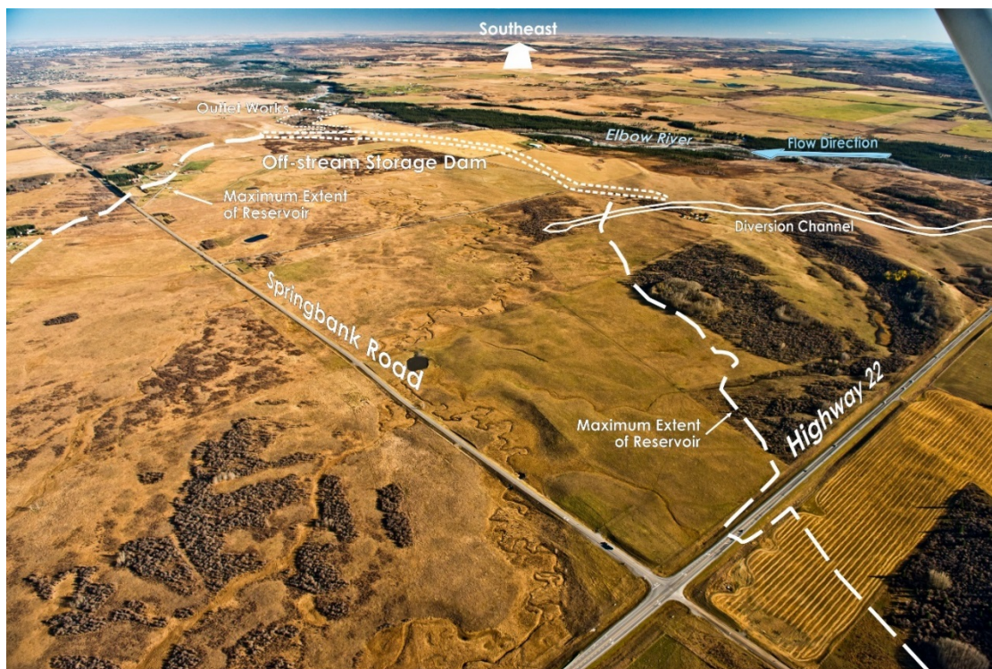
Figure 1-2 Looking Southeast towards the Off-Stream Reservoir and Dam
