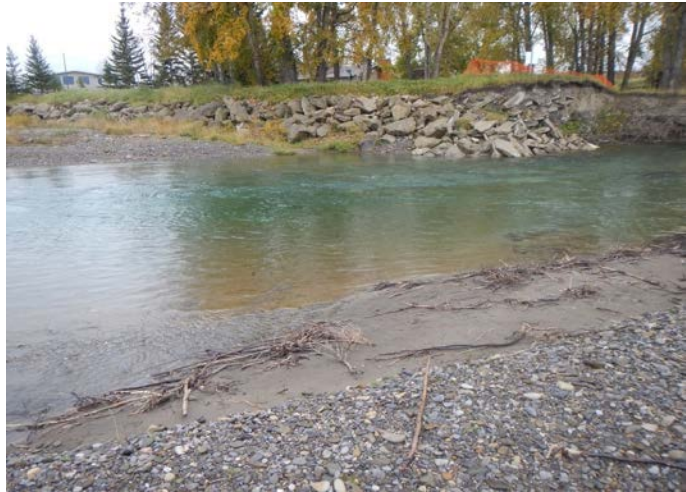
Photo 1: Downstream right bank from T1 with pool and artificial boulders.
