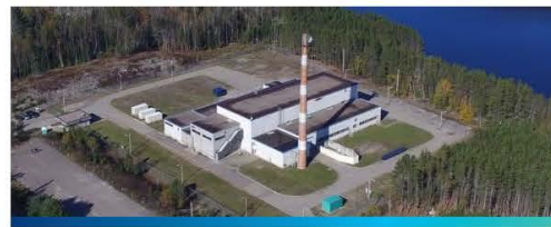
NPD Closure Project
