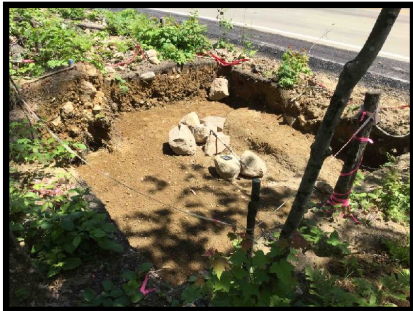
Photograph 14: Excavation at CaGi-67 Locale I
