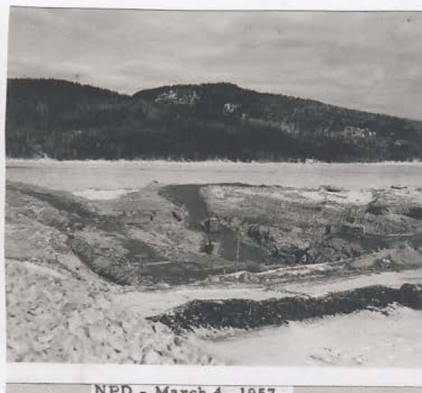
NPD - March 4, 1957 Figure 15c: Looking north at the excavation
