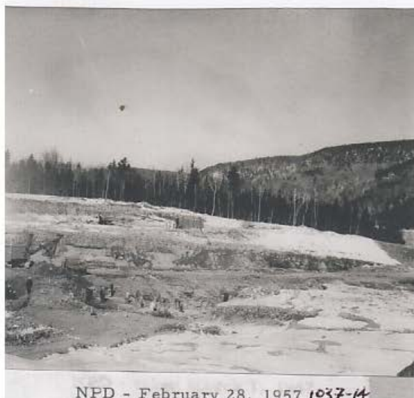
NPD - February 28, 1957 1037-14 Figure 15b: Looking northeast at the excavation
