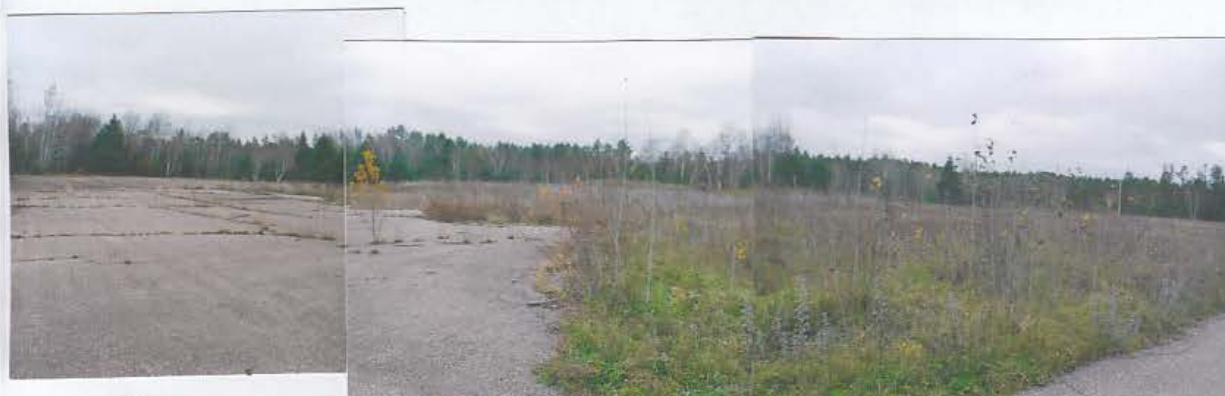
Figure 18b: Looking southeast over area of former training facilities
