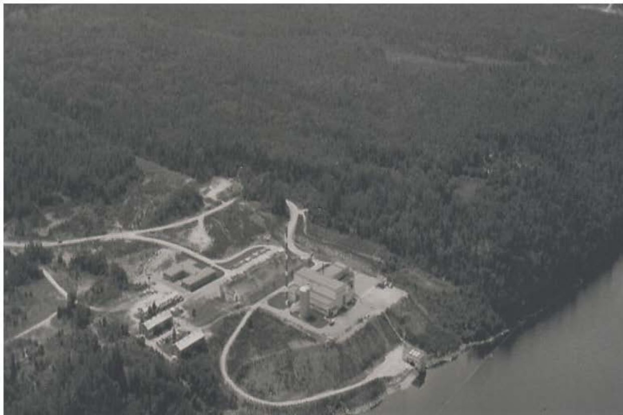
Figure 15a: Looking southeast over NPD shortly after construction
