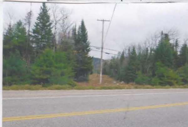
Figure 20e: Looking north down low voltage transmission line corridor
