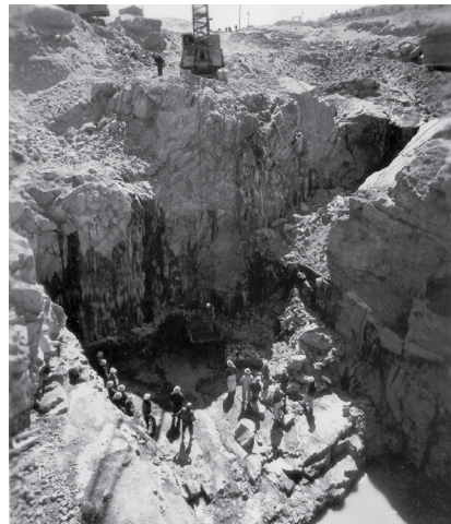
Bedrock excavated during the construction of NPD
