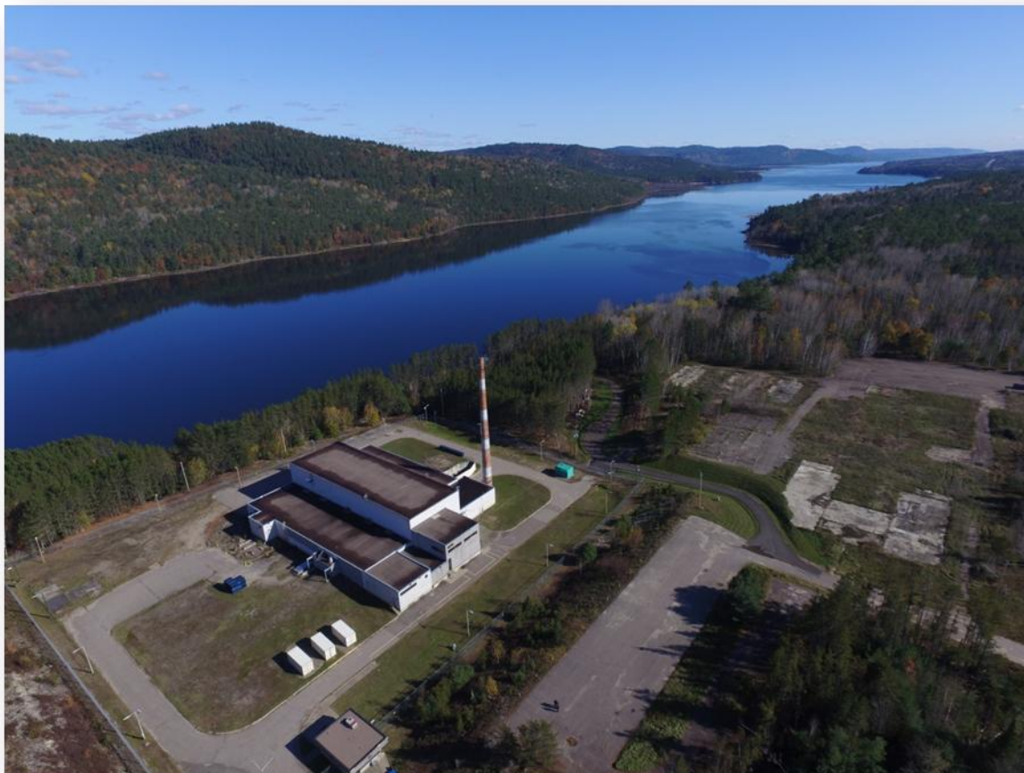
Figure 2-1 The Nuclear Power Demonstration Waste Facility.
