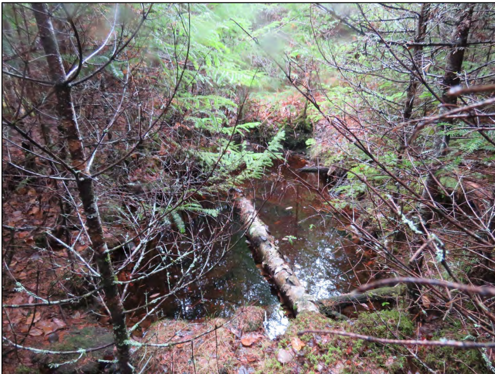
Plate 24: Overgrown geotechnical test pit, filled with standing water. Facing north; November 13, 2020.
