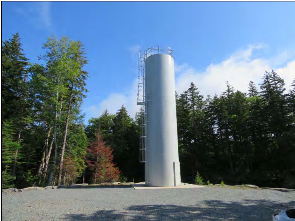
PLATE 4: Automated lime dosing station on the west bank of the Killag River. Facing northeast; July 22, 2019
