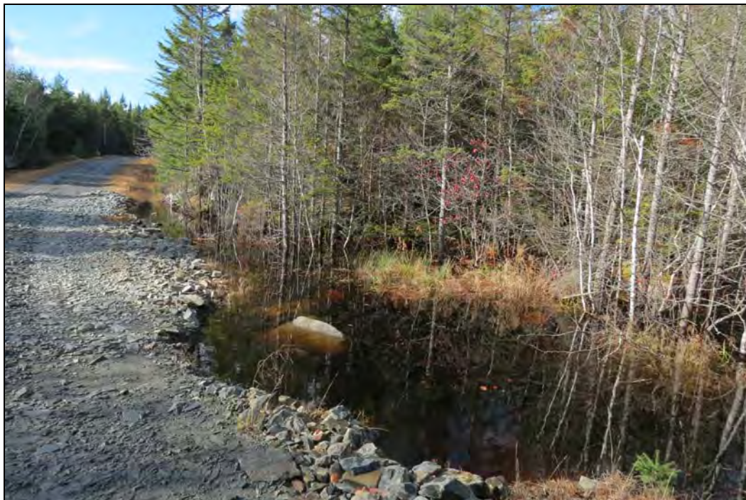
Plate 2: A flooded area along the proposed haul road; facing southeast. November 13, 2015.
