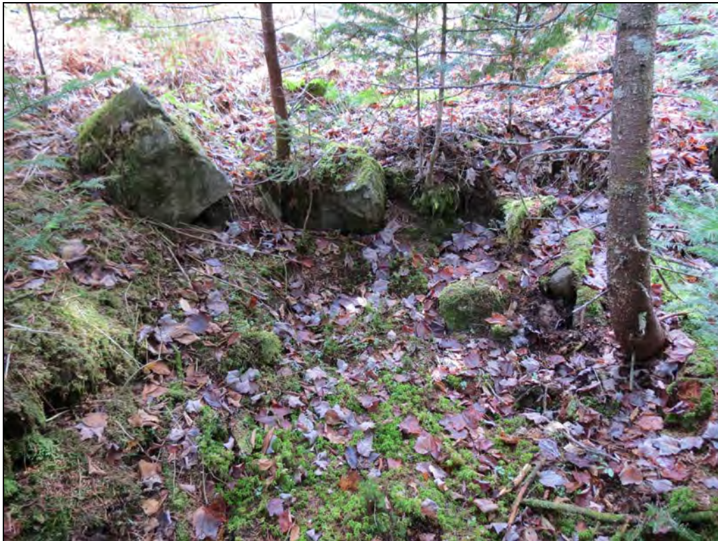
Plate 11: Possible tailrace along the north side of mill foundation; facing southwest. October 21, 2014.
