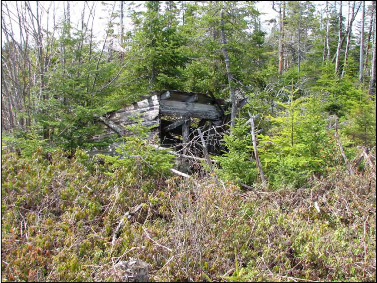
PLATE 13: Site 4: Remains of wooden structure; facing southeast.
