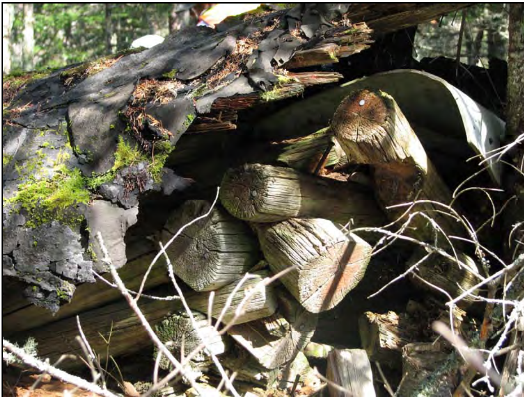
PLATE 9: Site 1: Detail of interlocking saddle notch corner construction technique.
