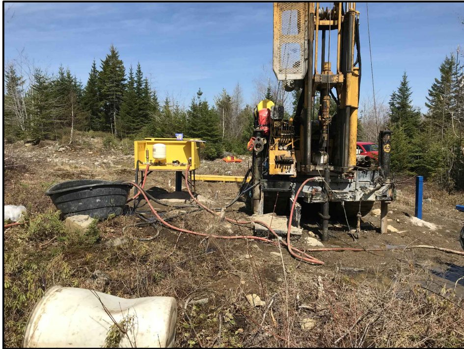
PHOTO 1 - DRILLING ACTIVITIES FOR BEAVER DAM MINE PROJECT
