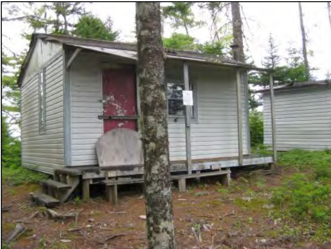
Looking northeast at the squatters camp "Cabin" building
