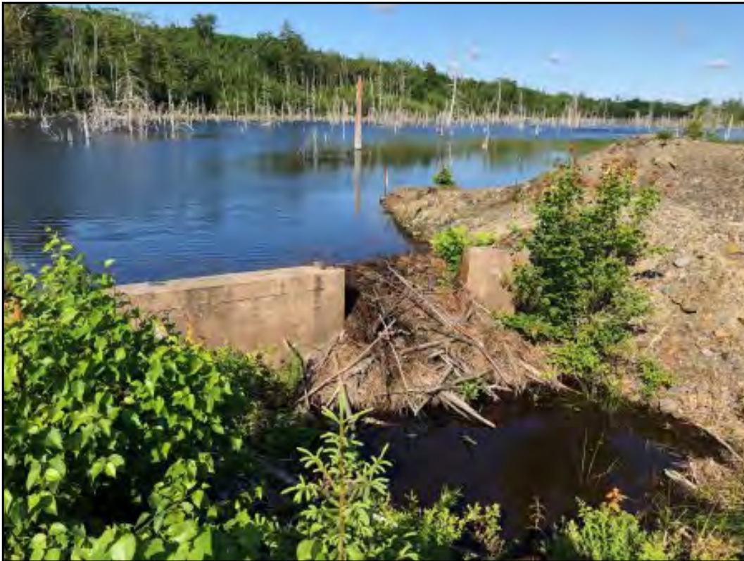
View of earthen dam spillway looking west
