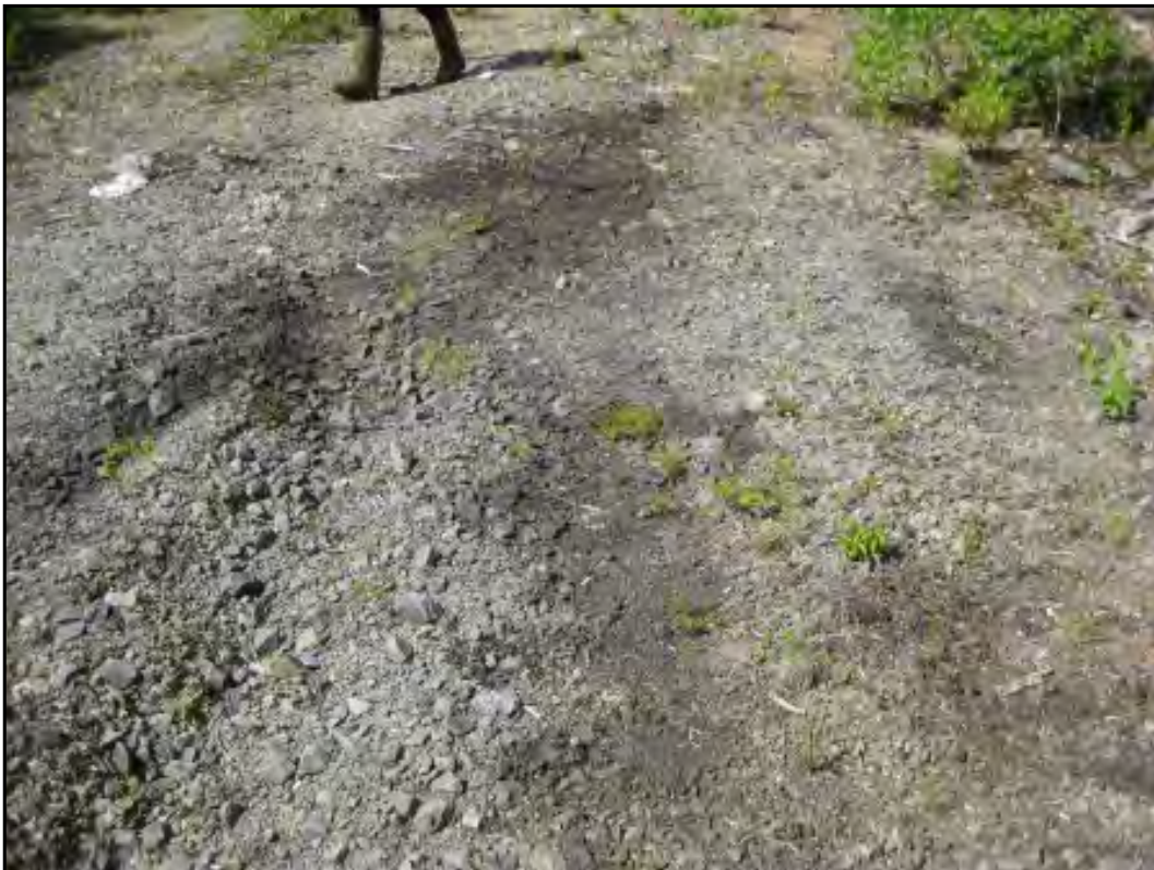
Typical example of small surface staining less than 2 sq.m. in various locations on the Site
