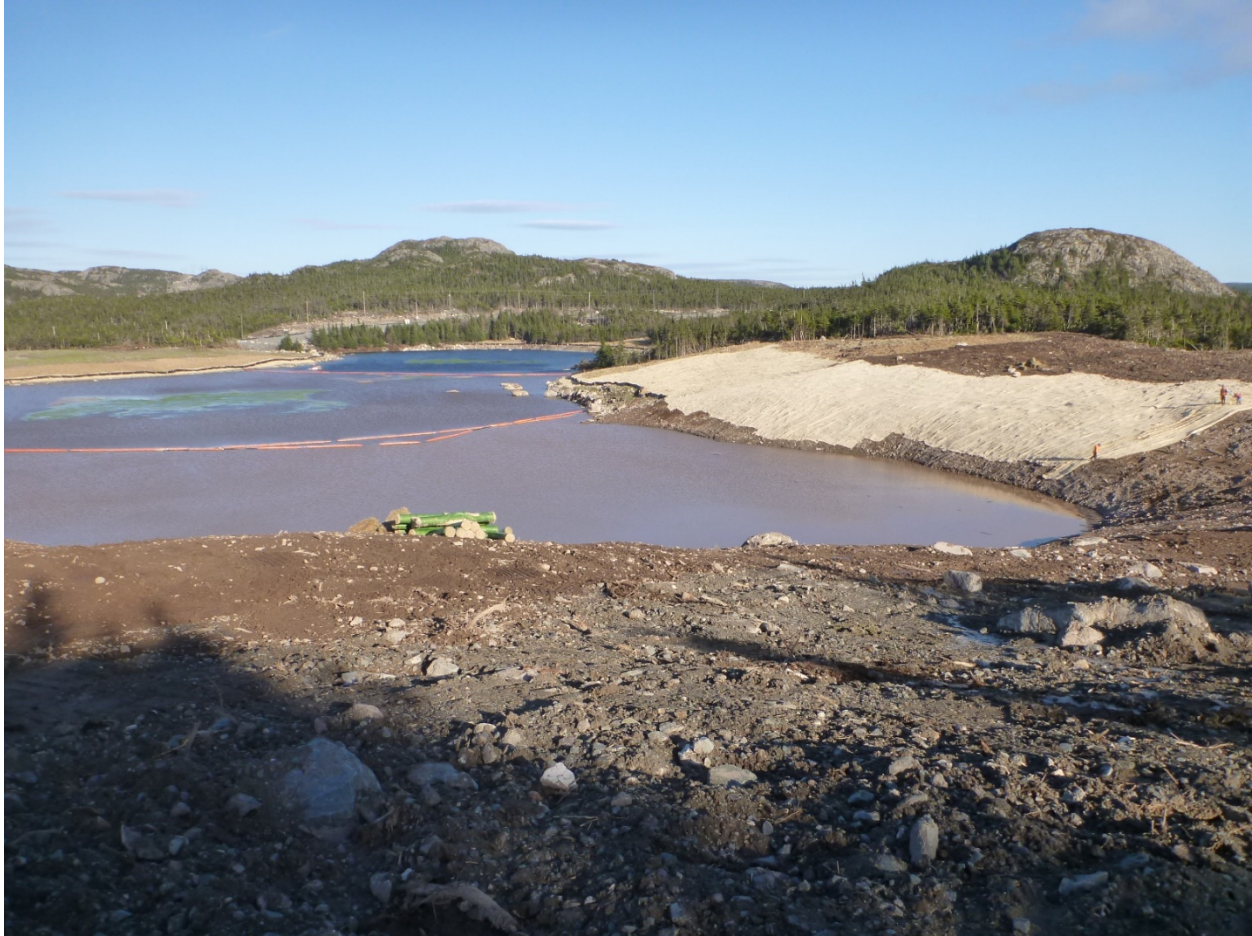
Figure 33: Typical large offset excavation to expand an existing waterbody
