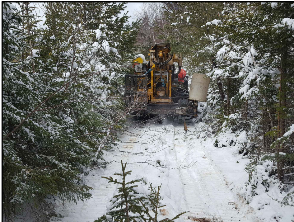
PHOTO 2 - DRILL RIG DURING MOBILIZATION TO "MW16"
