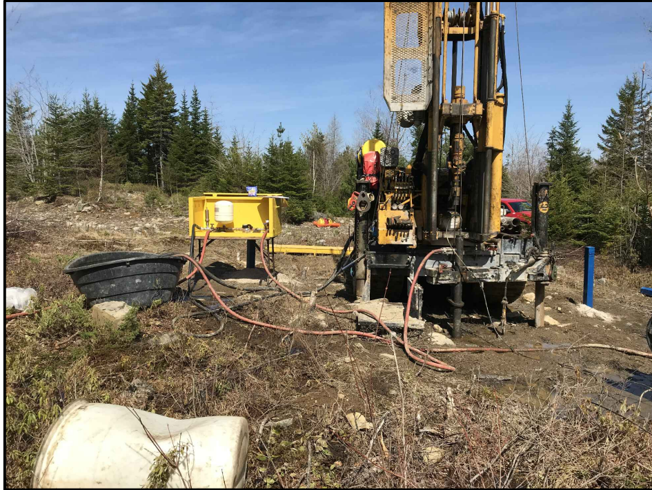
PHOTO 1 - DRILLING ACTIVITIES FOR BEAVER DAM MINE PROJECT
