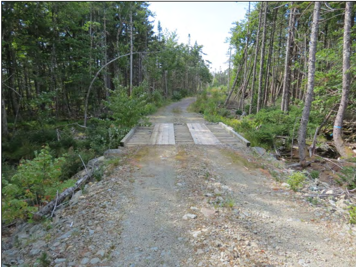
PLATE 9: Bridge crossing Middle Brook. Facing west; September 25, 2018.
