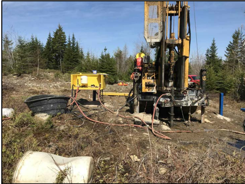
PHOTO 1 - DRILLING ACTIVITIES FOR BEAVER DAM MINE PROJECT
