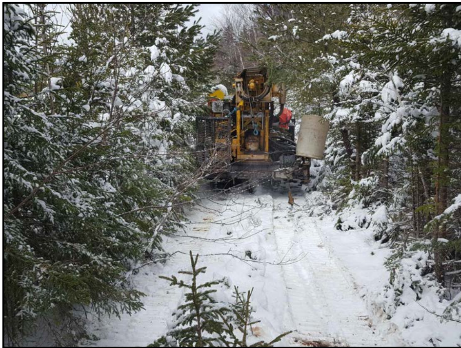
PHOTO 2 - DRILL RIG DURING MOBILIZATION TO "MW16"
