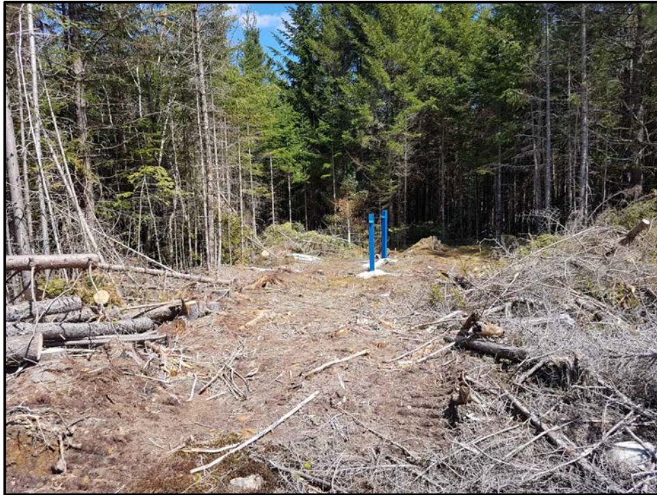
PHOTO 5 - VIEW OF STICKUP CASING FOR COMPLETED MONITORING WELLS "MW02"
