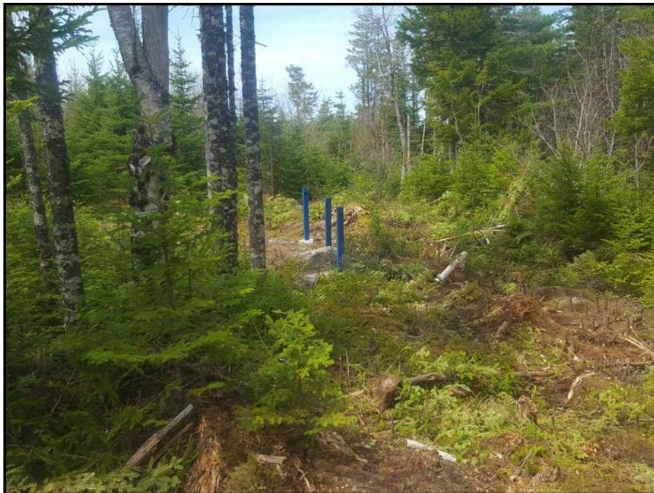
PHOTO 6 - VIEW OF STICKUP CASING FOR COMPLETED MONITORING WELLS "MW18"
