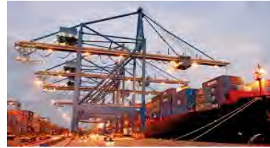
Quay Crane (QC)
