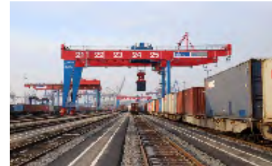
Rail Mounted Gantry Crane (Rail RMG)
