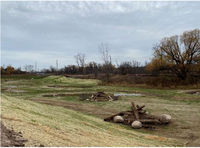
Photo 7: During construction Tributary A. South end of realignment. Off-line floodplain
