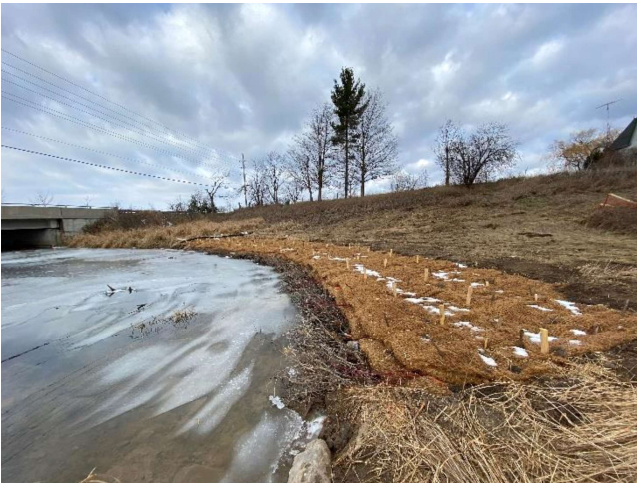
Photo 15: During construction Indian Creek (2022). Stabilized upstream right bank. Facing upstream (southwest)
