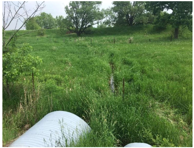
Photo 4: Pre-construction Tributary A (2020). At culverts under Tremaine Road facing upstream (north)
