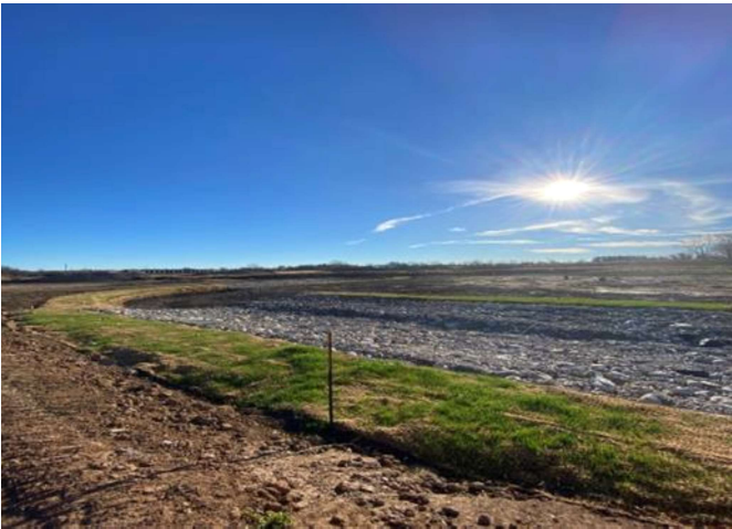
Photo 9: During construction Tributary A. Rock lined channel facing north.
