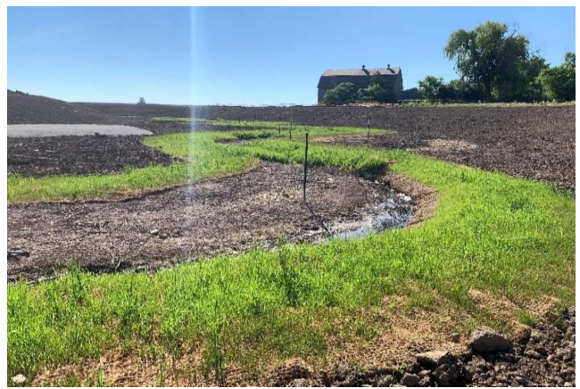
Photo 6: During construction Tributary A (2022). Downstream section facing downstream (southeast).
