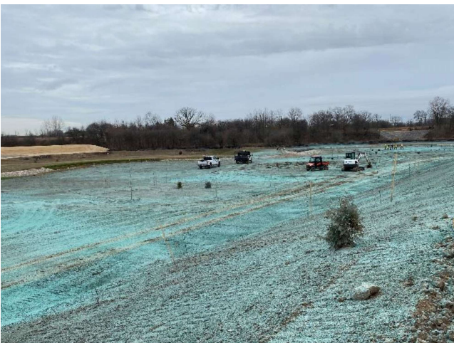
Photo 17: During construction Indian Creek floodplain (2022). Hydroseeding and tree planting
