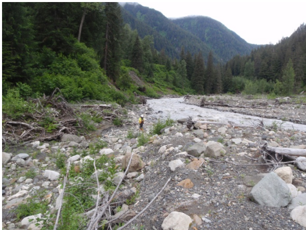
Photo 3: Looking downstream towards remnant flood channel and recent deposits of sediment & woody debris in the vicinity of Stn 5+200. June 13, 2017.
