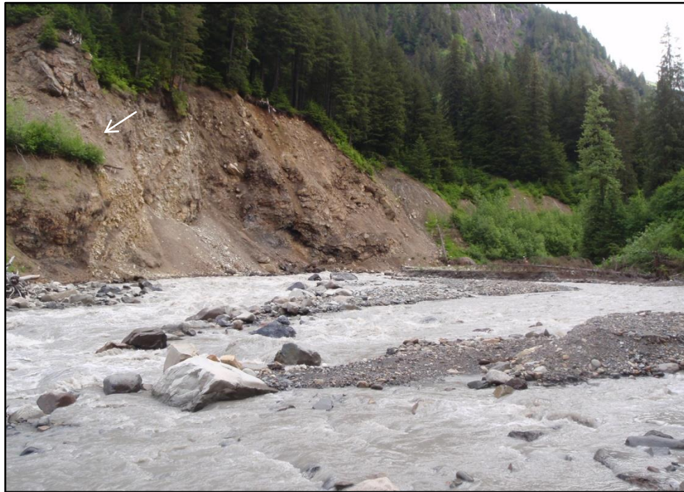
Figure 4-3 Looking upstream along the right bank of Bitter Creek towards the channel bend that is present between Stations 4+600 and 4+820. The Alders shown on the bank (see arrow) shows the location of the previously constructed road elevation.
