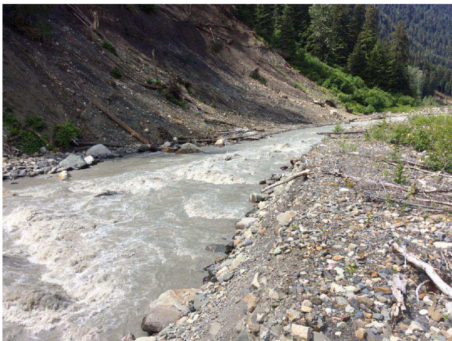
Figure 94. View from the north bank of Bitter Creek, near road station 3+220, looking downstream.
