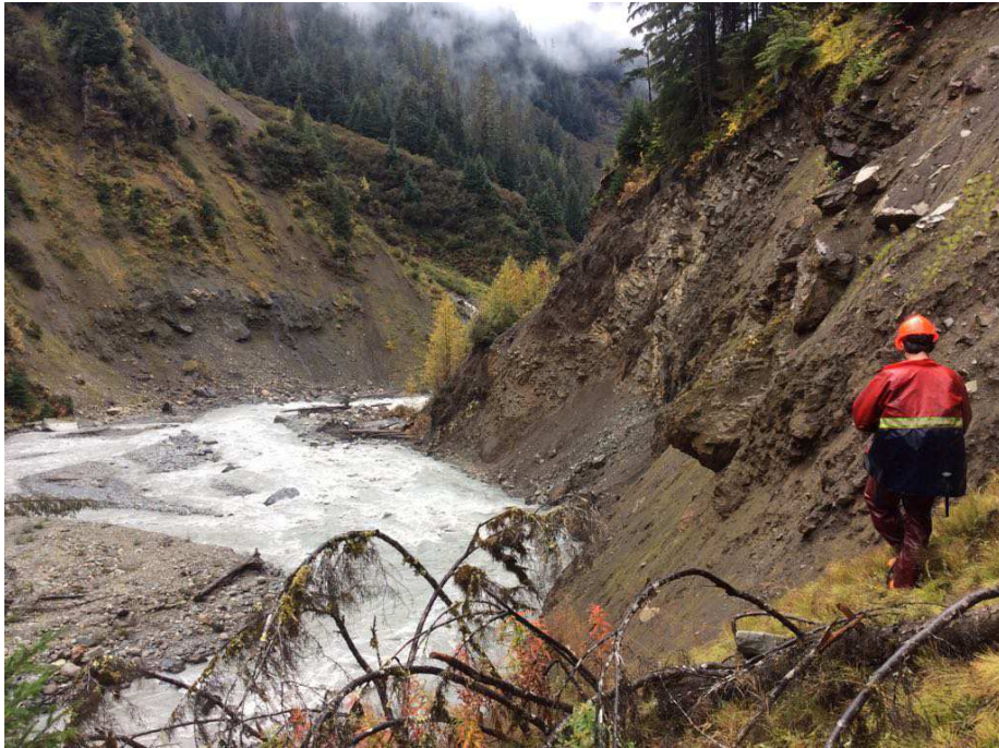
Figure 73. View from the north bank of Bitter Creek, near road station 4+765, looking downstream.
