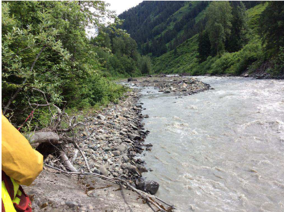
Figure 102. View from the north bank of Bitter Creek, near road station 3+490, looking upstream.
