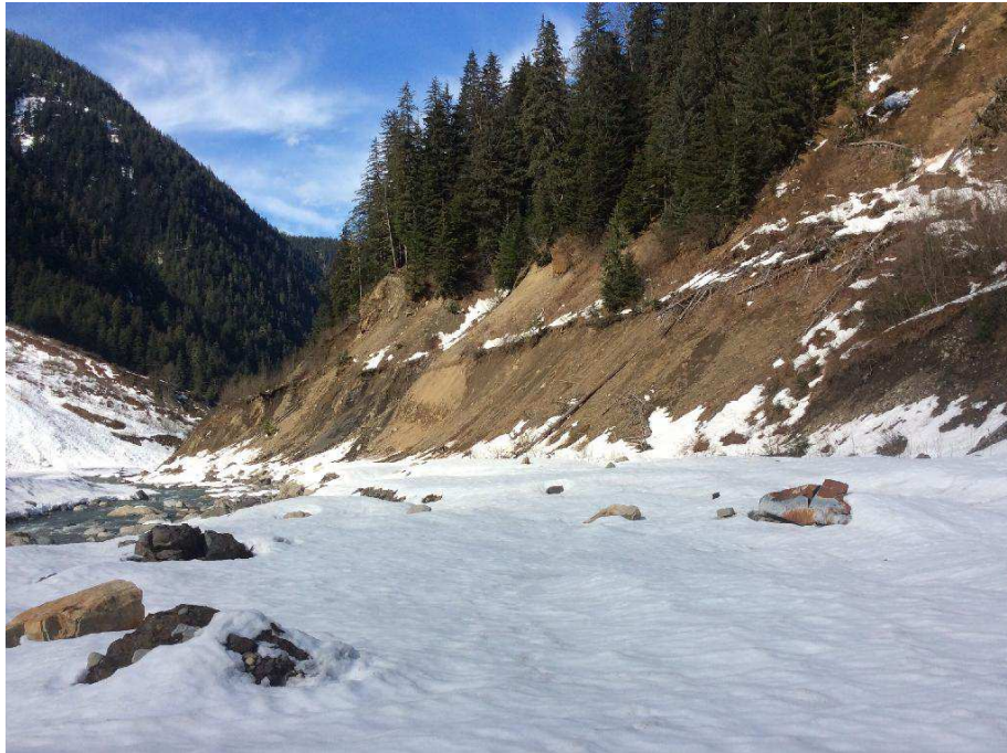
Figure 83. View from the north bank of Bitter Creek, near road station 4+450, looking downstream.
