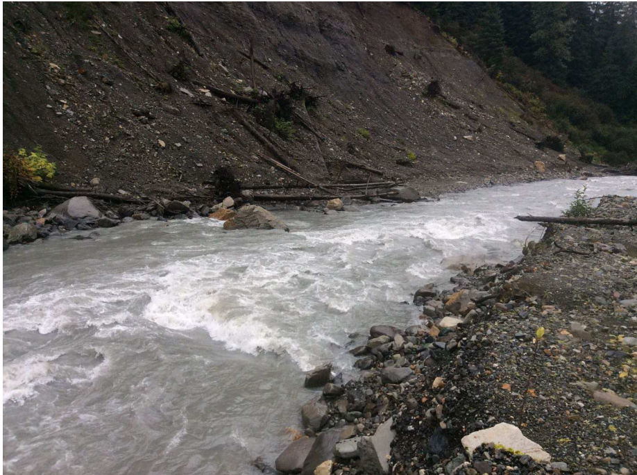
Figure 33. View of Bitter Creek near road station 3+210.
