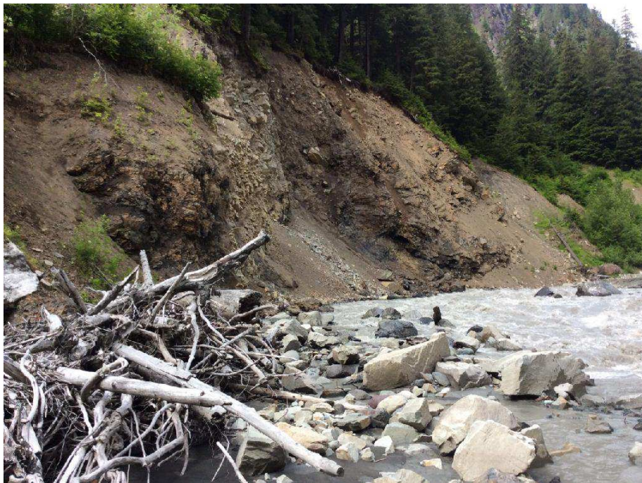
Figure 134. View from the north bank of Bitter Creek, near road station 4+630, looking upstream.
