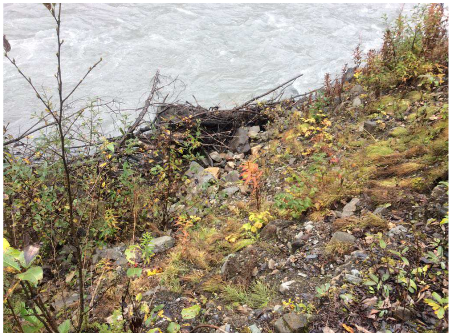
Figure 42. View of the north bank of Bitter Creek, near road station 3+450.
