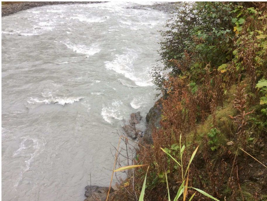
Figure 50. View of the north bank of Bitter Creek, near road station 3+990.
