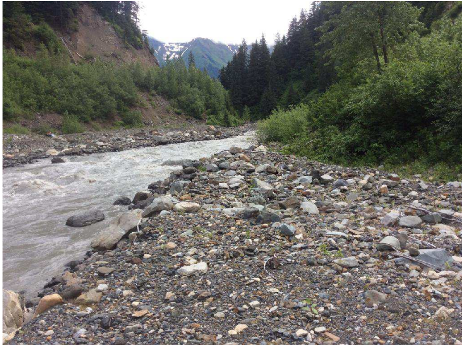
Figure 121. View from a gravel bar on the south side of Bitter Creek, near road station 4+400, looking upstream.
