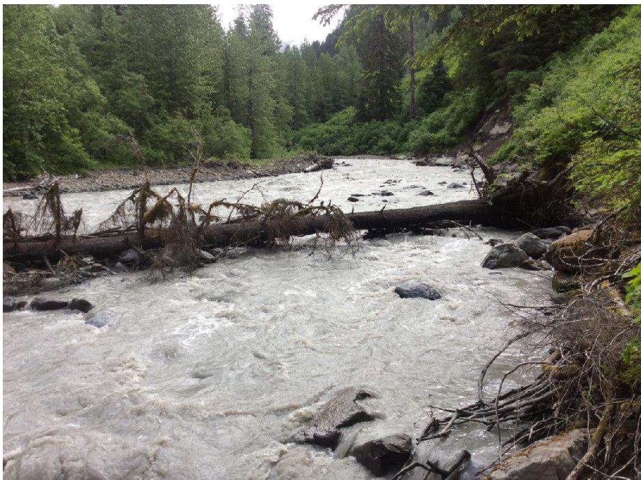
Figure 146. View from the south bank of Bitter creek, near road station 4+790, looking upstream.
