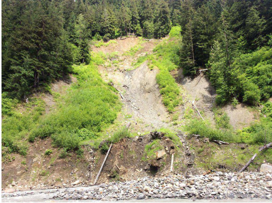
Figure 111. View from the south bank of Bitter Creek, near road station 4+065, toward the slope failure on the north bank.
